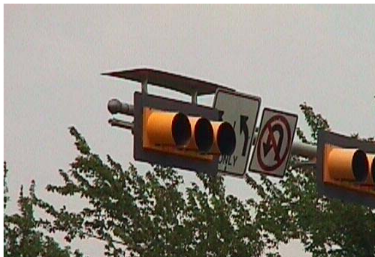
Figure 39. Texas Flat Panel Damper.
