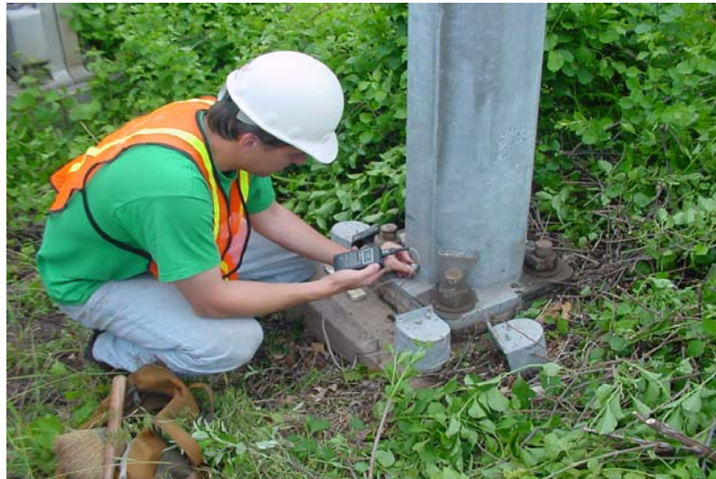
Figure 32. Thickness Measurement at Critical Location of Structure Post.
