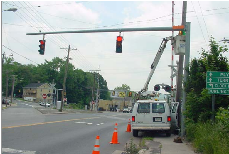
Figure 26. Inspection of a Mast Arm Structure.
