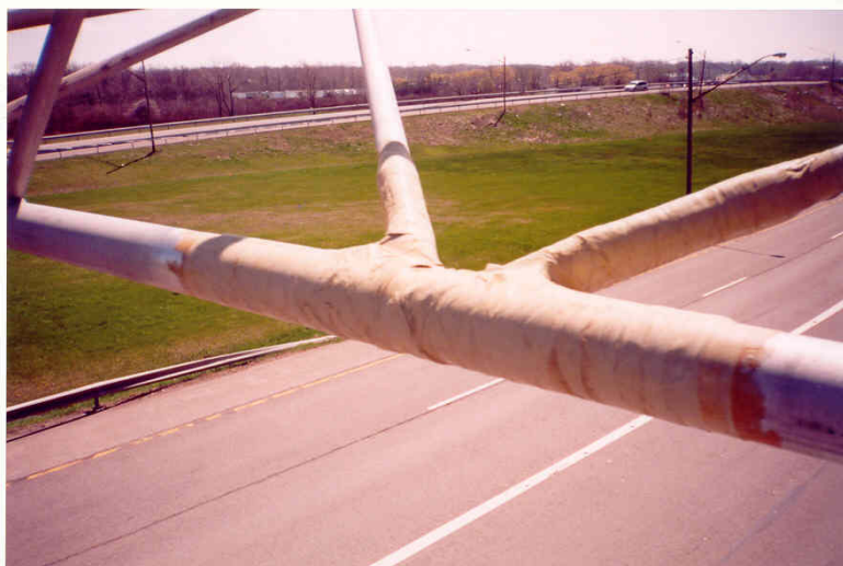
Figure 37. Repair of Truss Members Using FRP.
