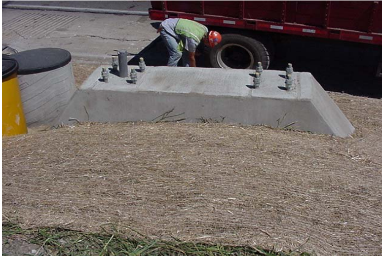
Figure 5. Foundation Ready for Structure Installation.
