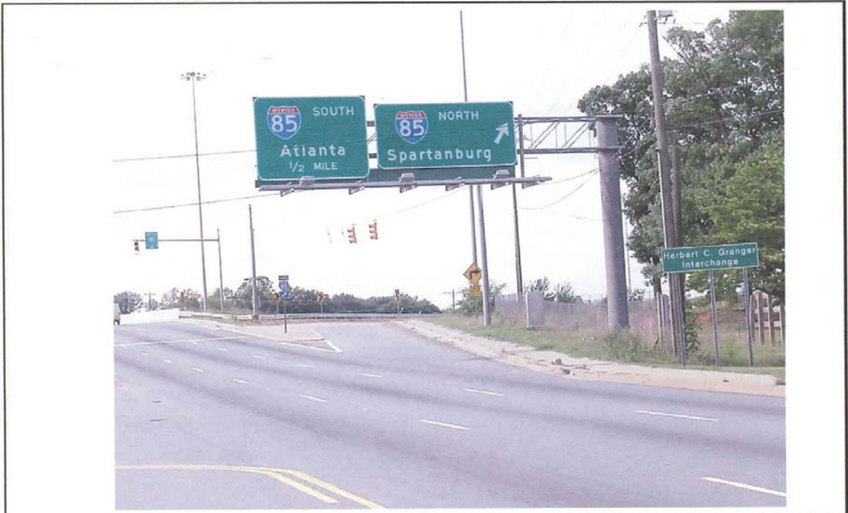
PHOTOGRAPH 1: FRONT OF STRUCTURE
