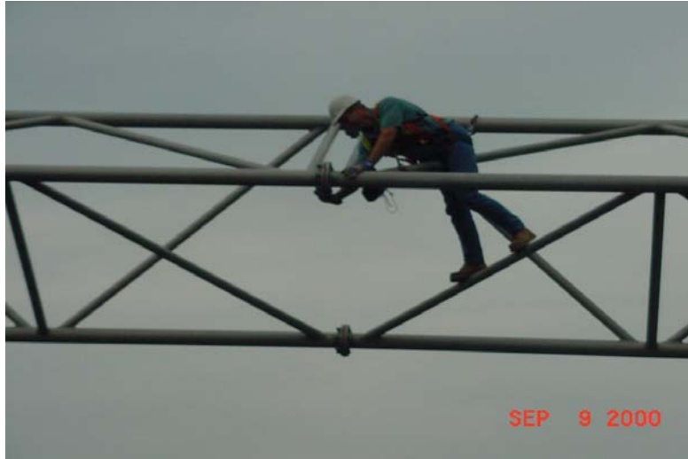
Figure 25. Hands on Inspection of Overhead Signs.
