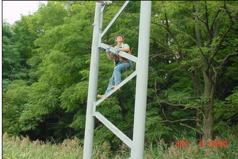
Figure 17. Inspector Climbing Structure.
