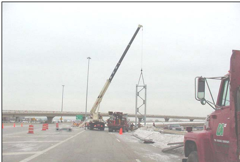
Figure 6. End Frame Being Set Onto Its Foundation.
