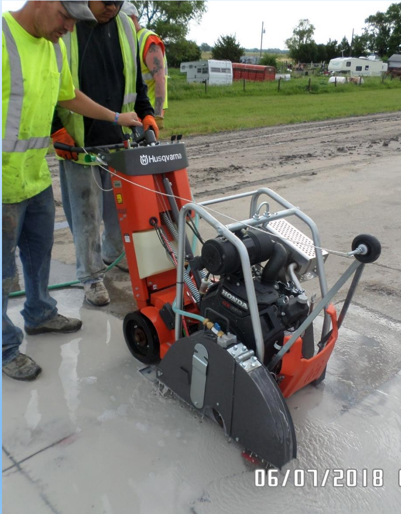
Sawing Pavement
