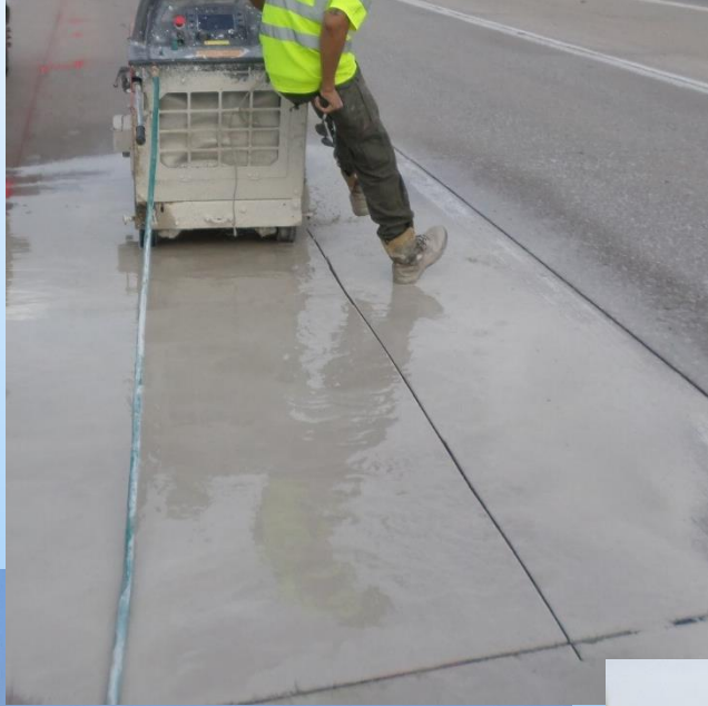
Sawing Pavement
