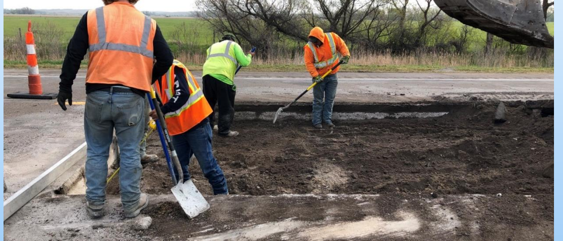
Remove small debris and level the base
