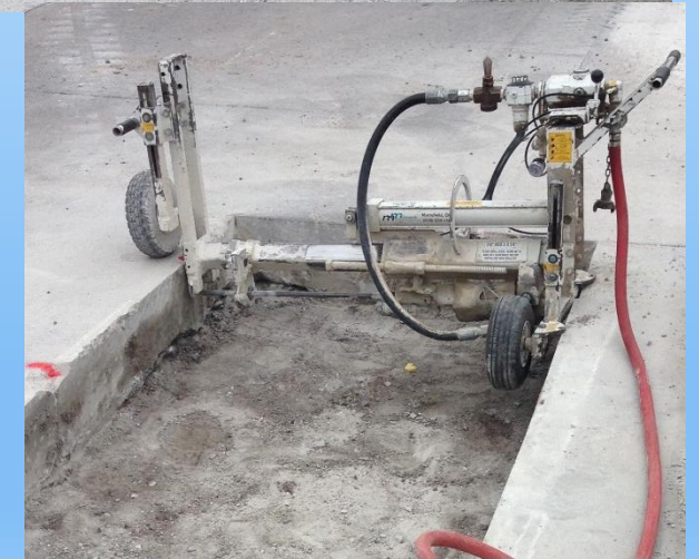
Drill used for holes- minimum opening size is 4 ft.
