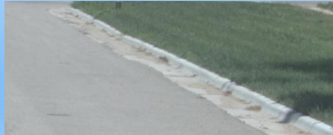
Combination Curb and Gutter
