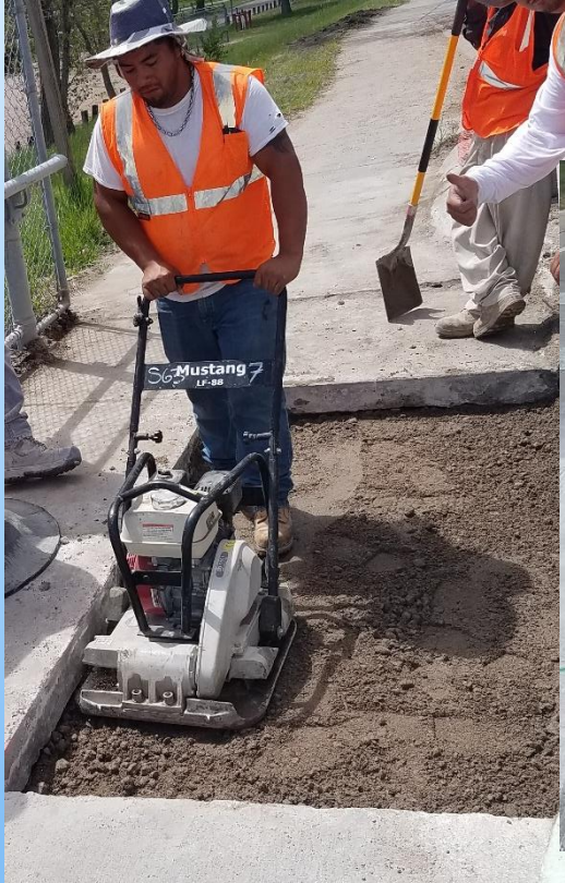
Preparation of base with dynamic plate compactor
