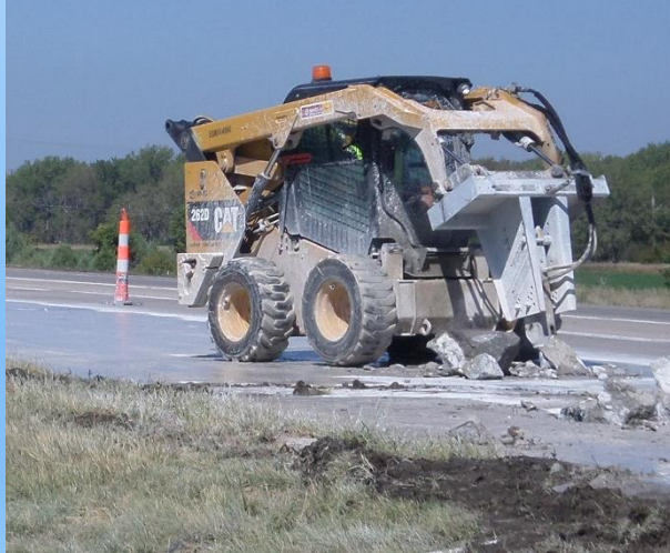
Skid loader with breaker
