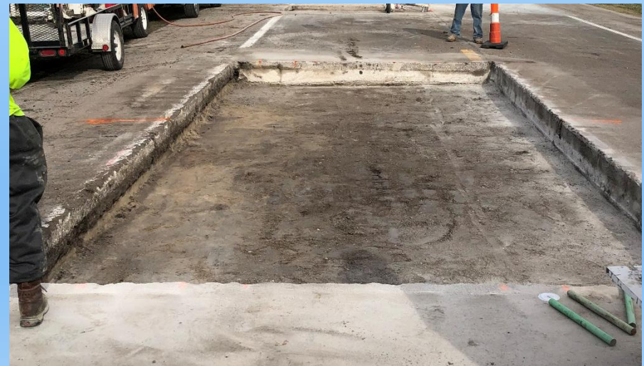
Leveled and compacted base
