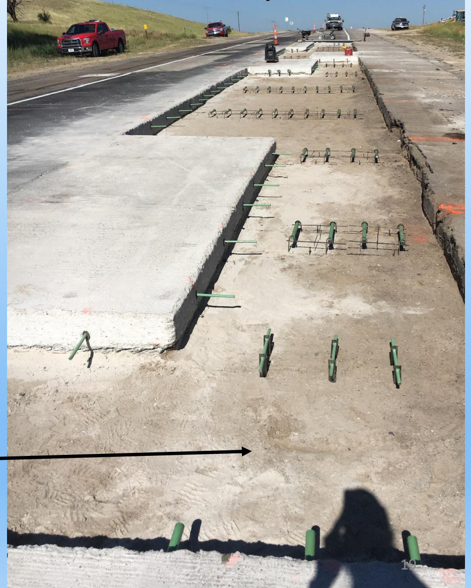
Subgrade is prepared for concrete repairs.
