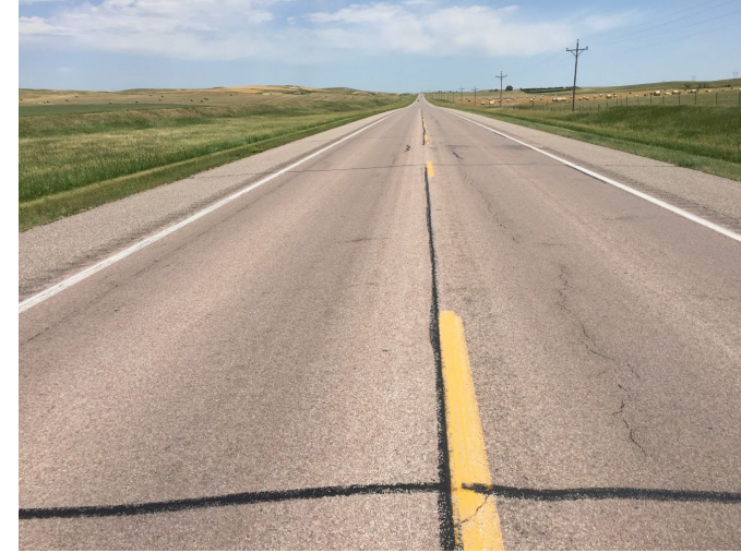
Crack seal in Nebraska
