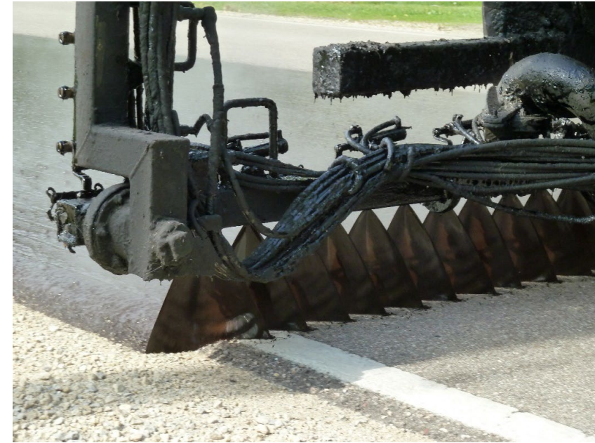
Chip seal asphalt emulsion in Wisconsin
