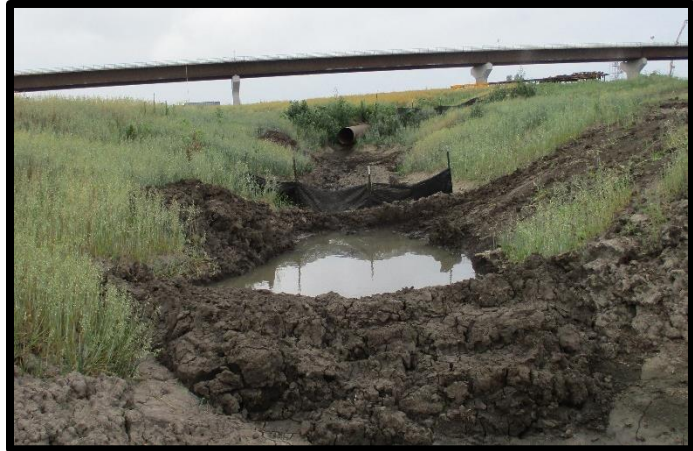
Figure 3: Silt traps are used in conjunction with other BMPs to help reduce sediment load and slow flow paths.
