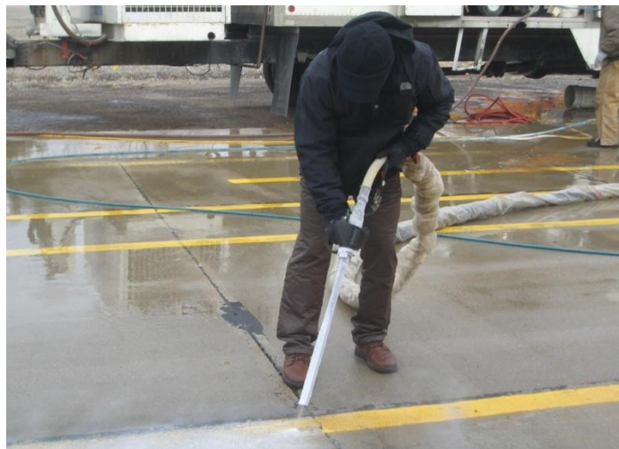
Figure 6.6. Dry ice is shot onto the markings
