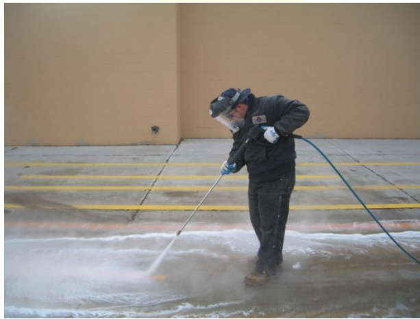
Figure 6.17. Operator with proper protection while removing marking by chemical method
