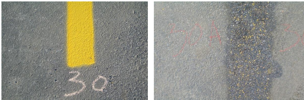
Figure 6.9. Asphalt pavement condition before (left) and after (right) paint has been removed by dry ice blasting
