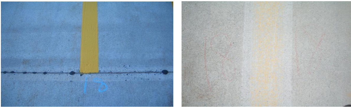
Figure 6.12. Concrete pavement condition before (left) and after (right) paint has been removed with scarifier
