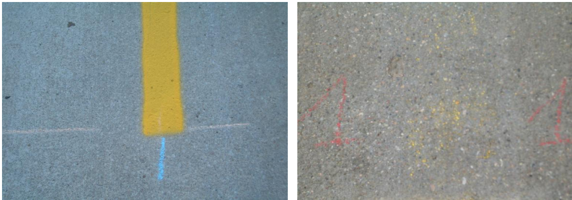
Figure 6.1. Concrete pavement condition before (left) and after (right) 12 mils water-based paint has been removed by water blasting
