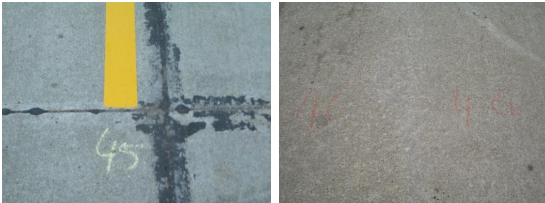
Figure 6.4. Concrete pavement condition before (left) and after (right) tape has been removed by water blasting
