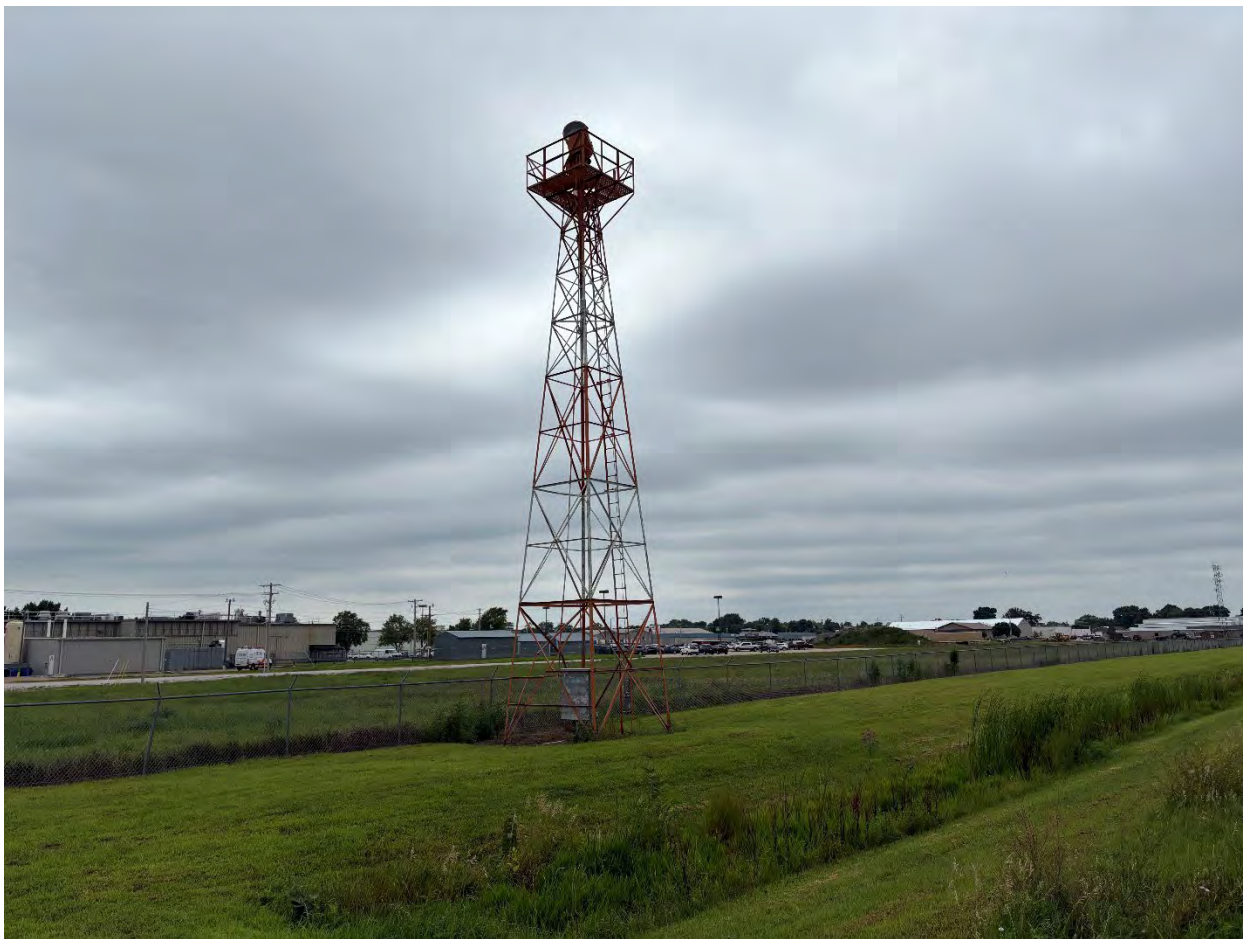
Existing beacon tower.
