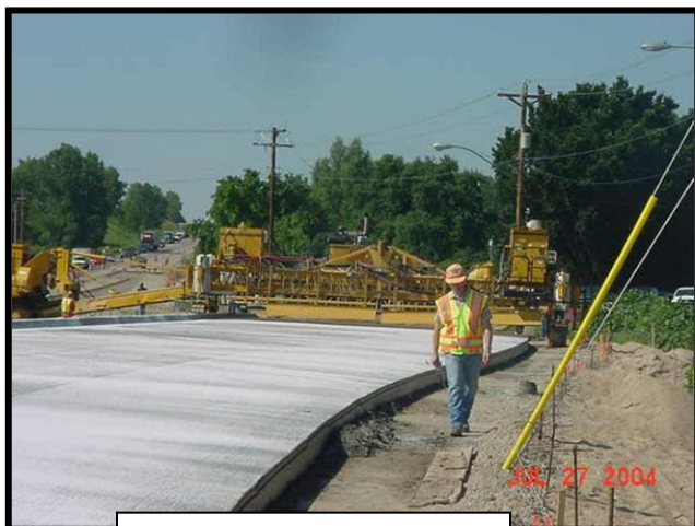
Paving Operation Finish
