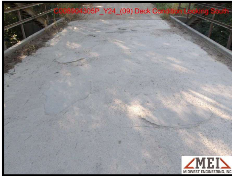
Photo 2: 2024 Deck Surface With Large Failing Patches
