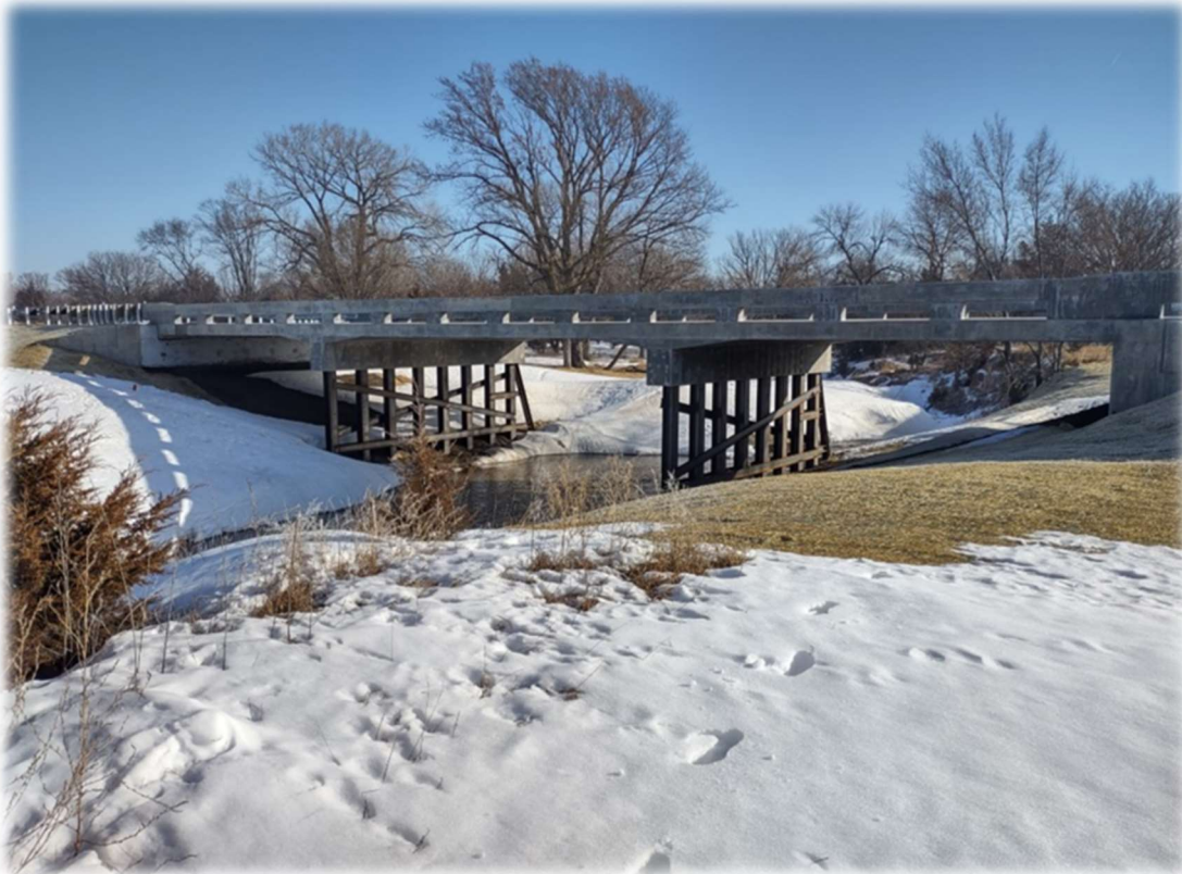
3-Span Continuous Concrete Slab Bridge (example).
