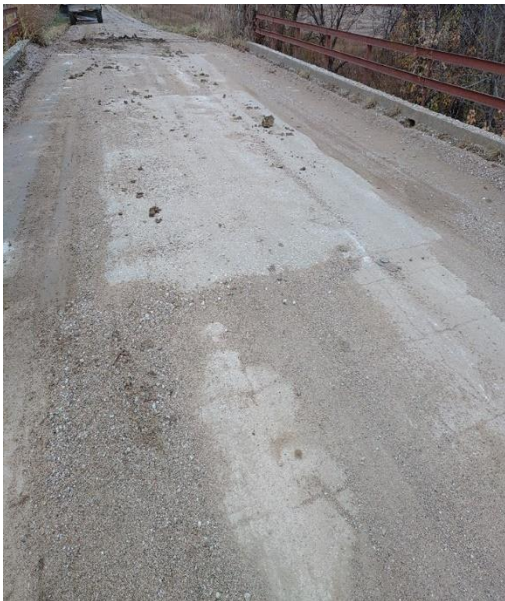
Figure 1: Concrete repair on 30% Deck
