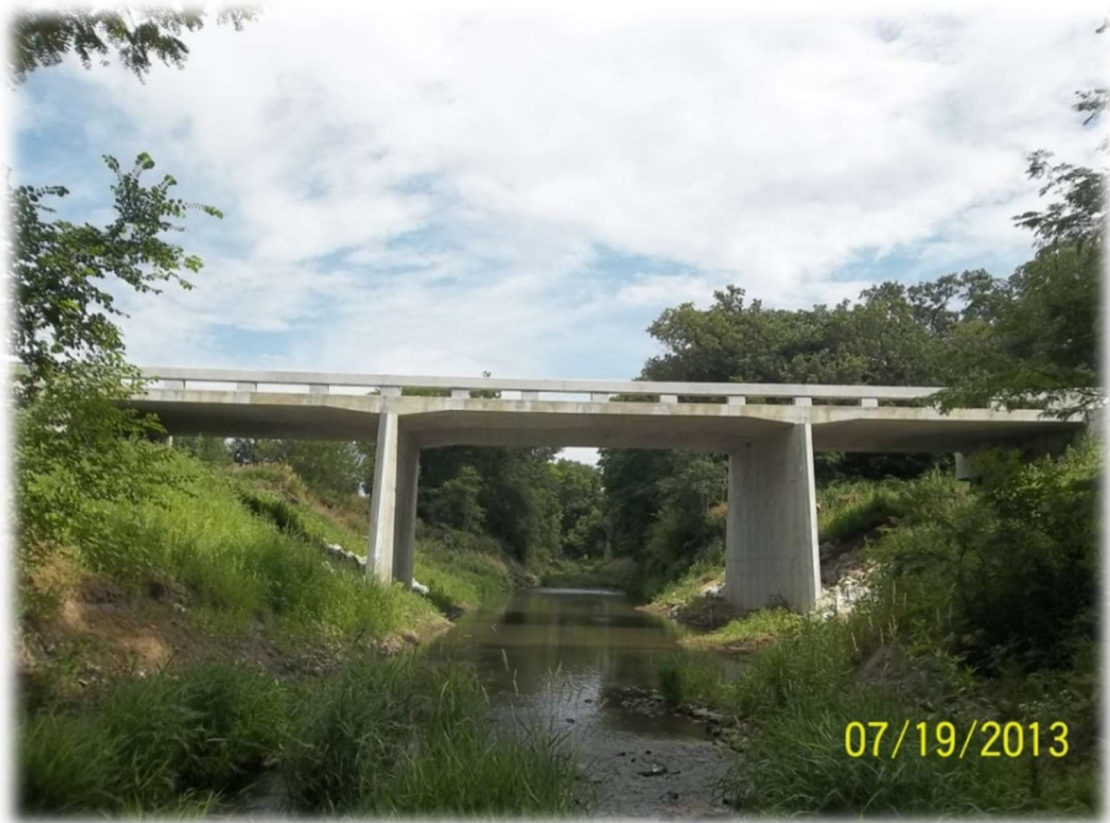
Continuous Concrete Slab Bridge (example).
