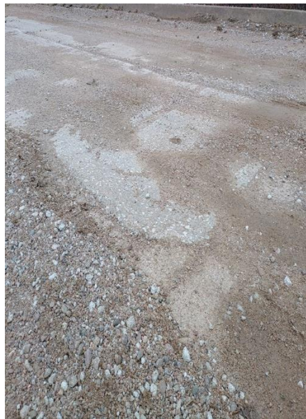
Figure 2: Top of recent deck patch, Abutment 2
