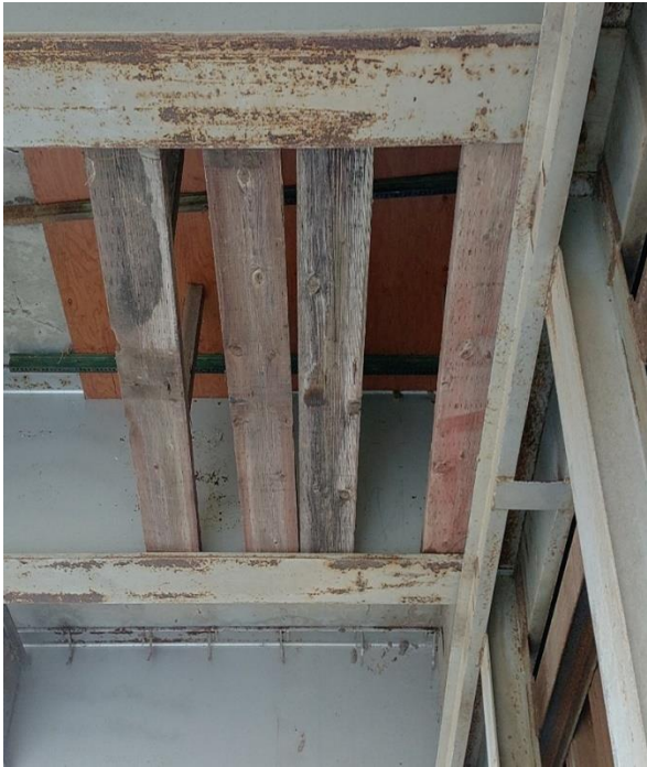
Figure 6: Cribbing between Girders 2 & 3
