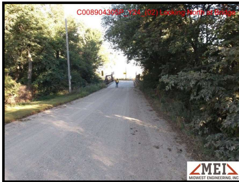
Photo 5: Looking North at Bridge and Alignment
