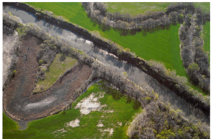
FIGURE 4: Meandering loops of Salt Creek northwest of Waverly were cut through to straighten the channel where Bridge G-222 will be reconstructed.
