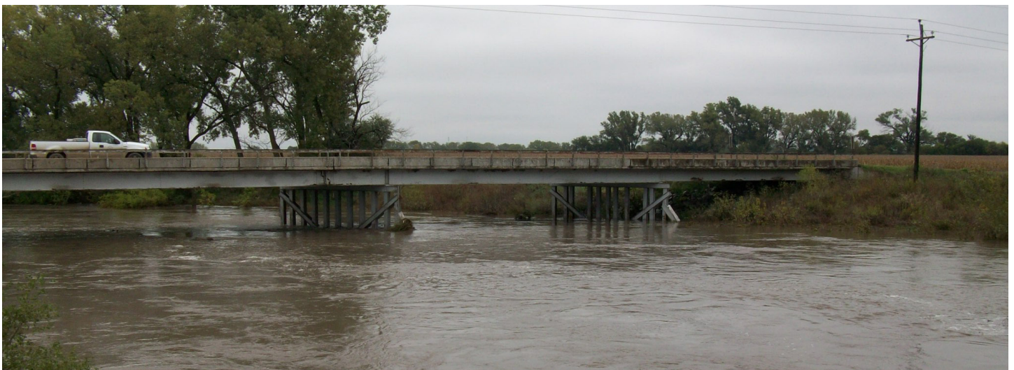
FIGURE 6: The current bridge location passes stream flows that are significantly influence by upstream channelization and flood control levees through Lincoln. The new bridge will safely pass the 100-year flood flows as Lincoln continues to grow.
