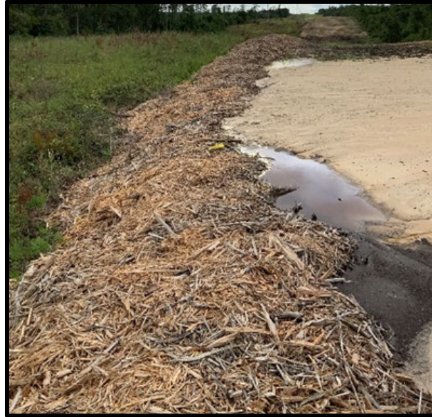
Figure 3.5 Slash Mulch Berm Installation in Alabama (photo courtesy of C. Young 2021)
