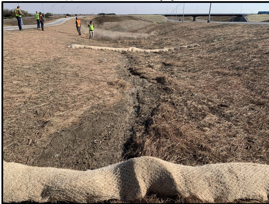
(b) wattle silt check as ditch protection
