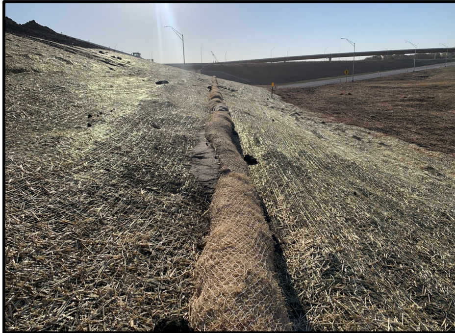
(a) wattle silt check as slope protection
