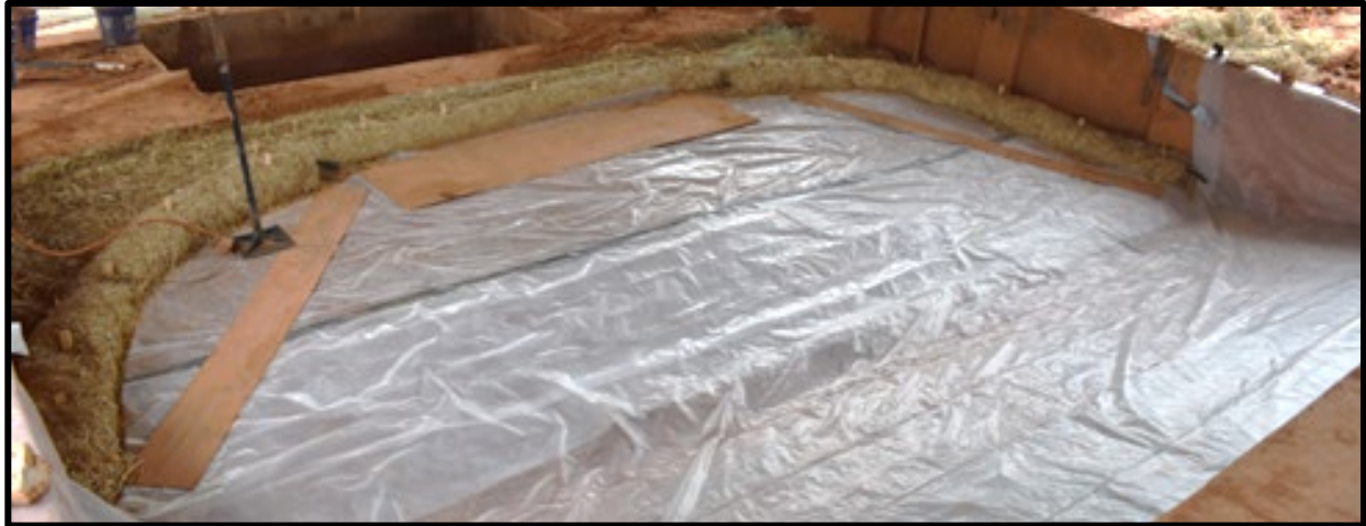
(a) straw wattle silt check standard installation
