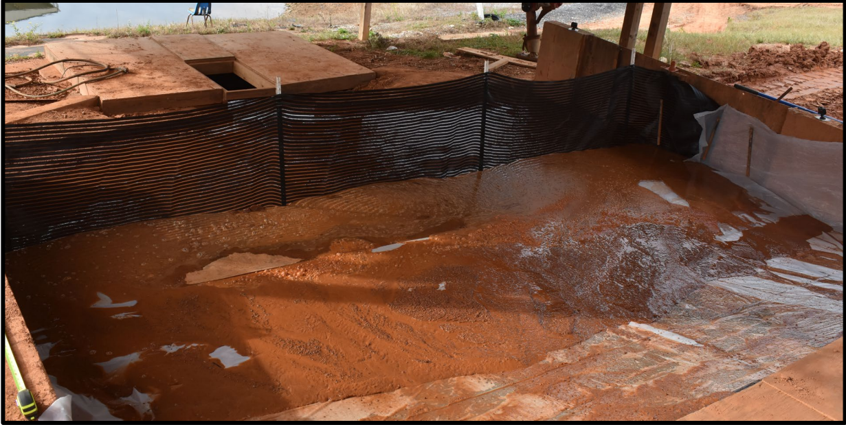
Figure 3.18 Performance of High Porosity Silt Fence Installation
