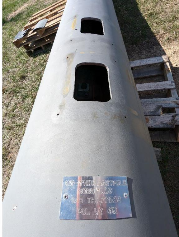
Figure 7.7 Two 5"x7" unreinforced access holes (courtesy of WYDOT)
