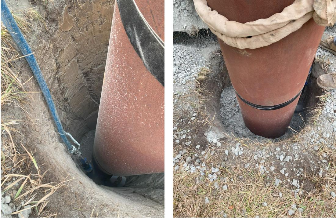
Figure F.2 Gravel backfill is used to fill the drilled holes with a pneumatic tamper to ensure uniformly compacted around the annulus
