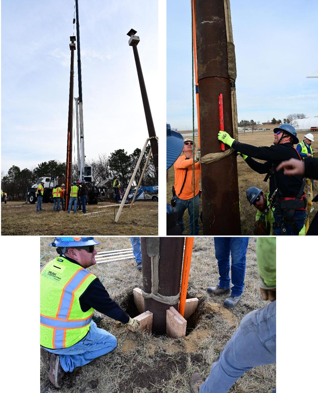
Figure 3.11 Installing the pole vertically in the pole and make sure it is installed at the center
