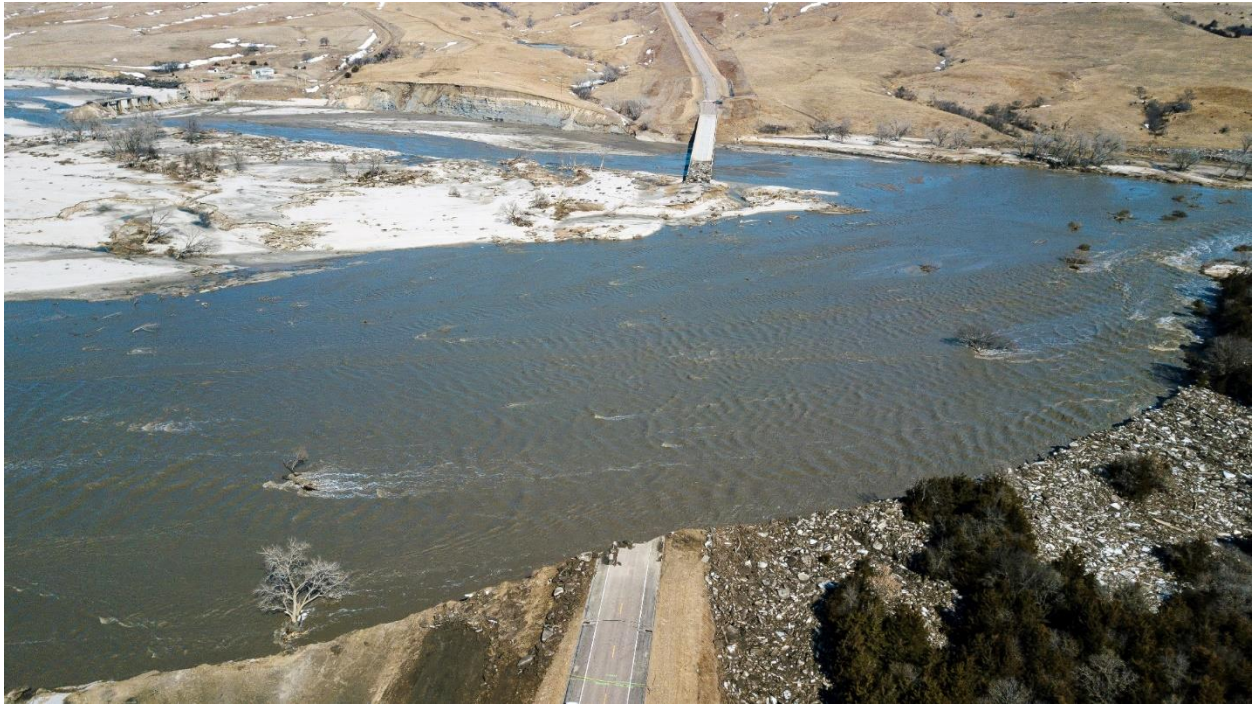
US-281 Bridge over Niobrara River, NDOT, March 2019
