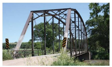
the traveling public with a crossing of Verdigre Creek in the vicinity of the existing crossing on 885 Road. This project is needed because the existing bridge is substandard in width, has deteriorated, and is near the end of its useful life. Additionally, the current alignment of 885 Road with the bridge does not meet minimum design standards.
