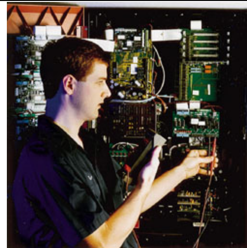
SimplexGrinnell Technicians Have Extensive Experience in the Fire Protection Industry.
