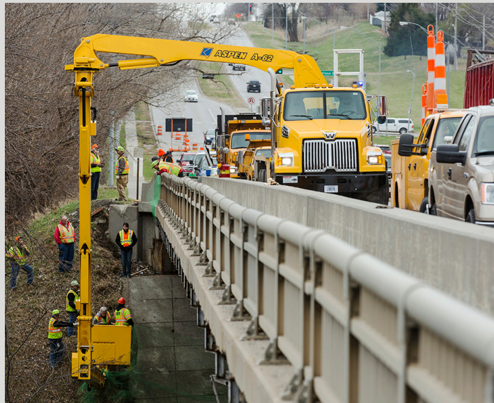
Bridge inspections are completed in accordance with National Bridge Inspection Standards (NBIS).
