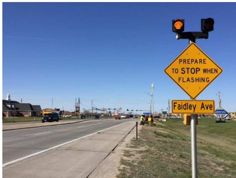
Figure 2.1 Advance Warning System (AWS) assembly on NB 281 in Grand Island, NE
