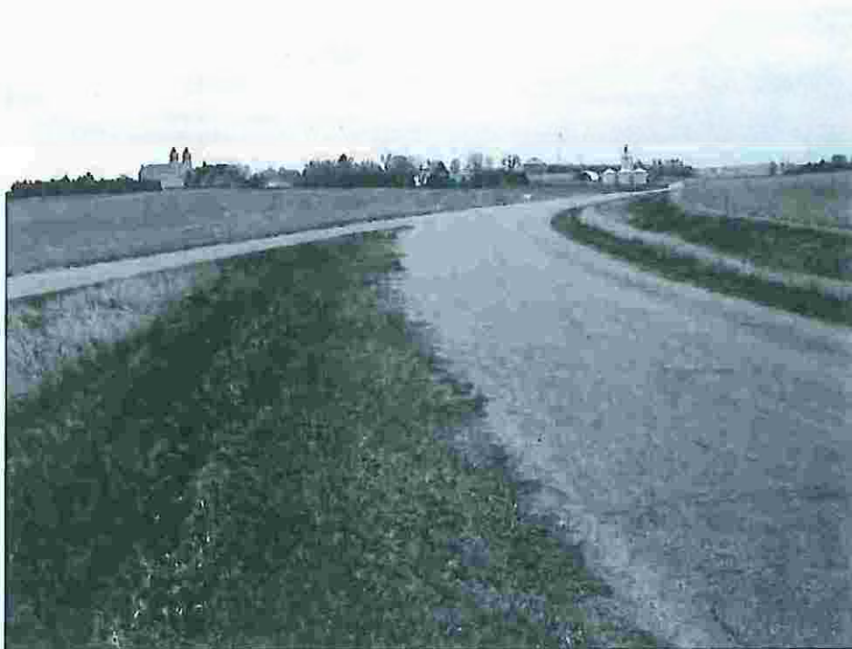
Photo #6245 1 ½ miles exiting curve, looking south-southeast.
