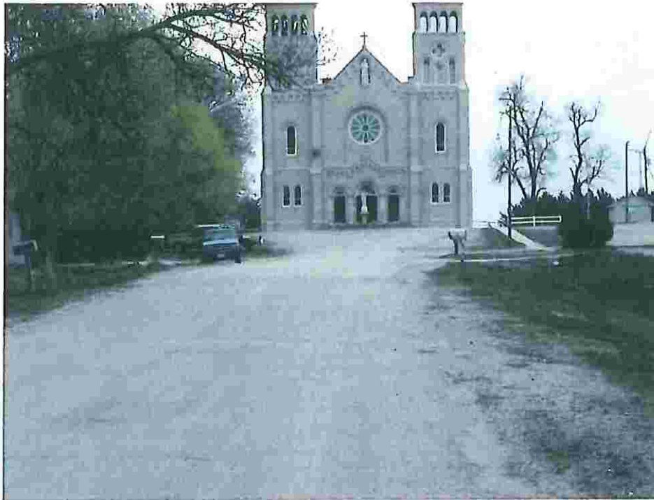
Photo #6251 After intersection Main Street and West R Road looking east.
