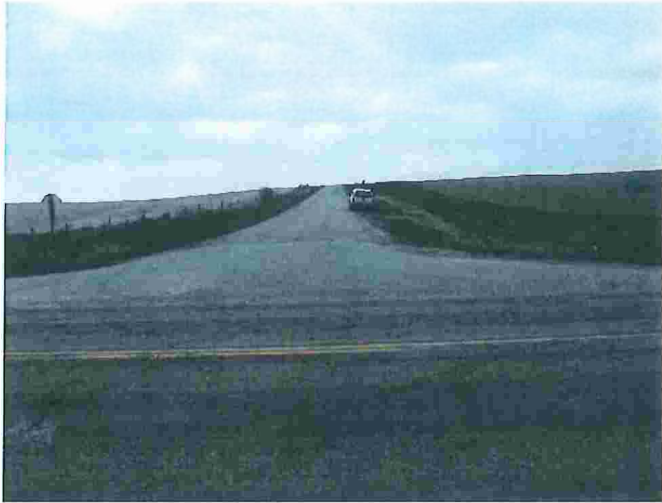
Photo #6234 West end of project looking east.
