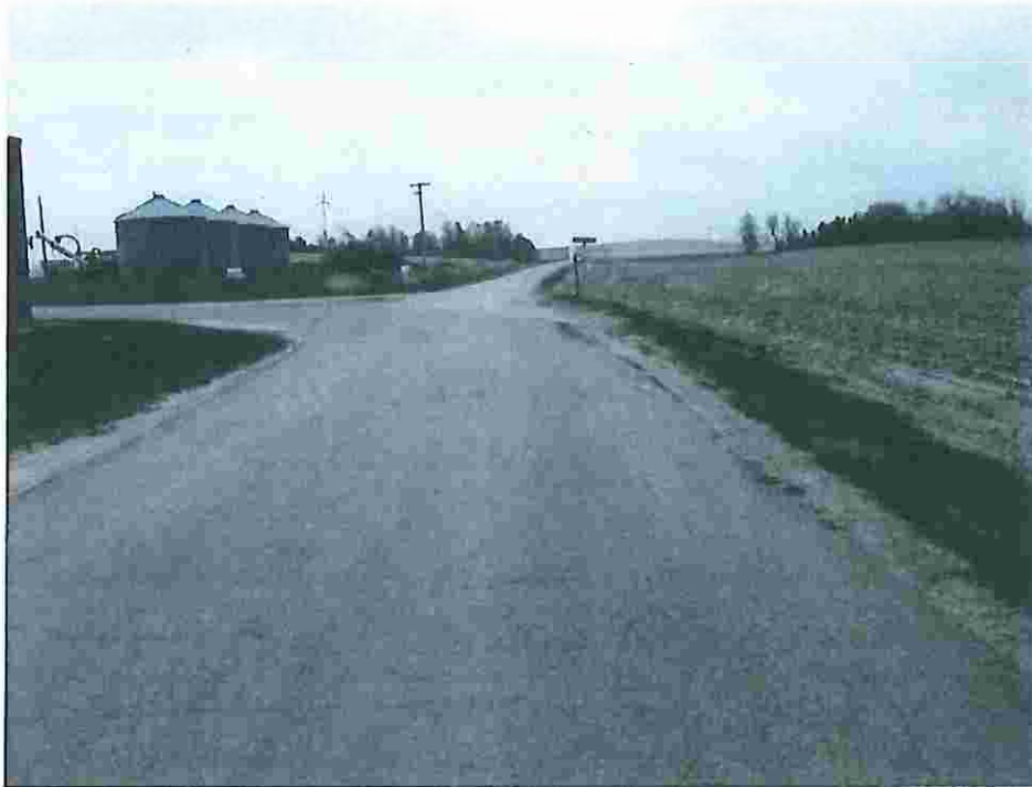
Photo #6247 Corner into Raeville looking south.
