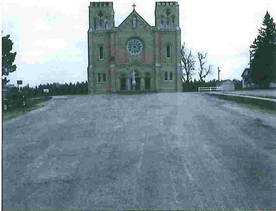
Photo #6253 East end of project looking east.
