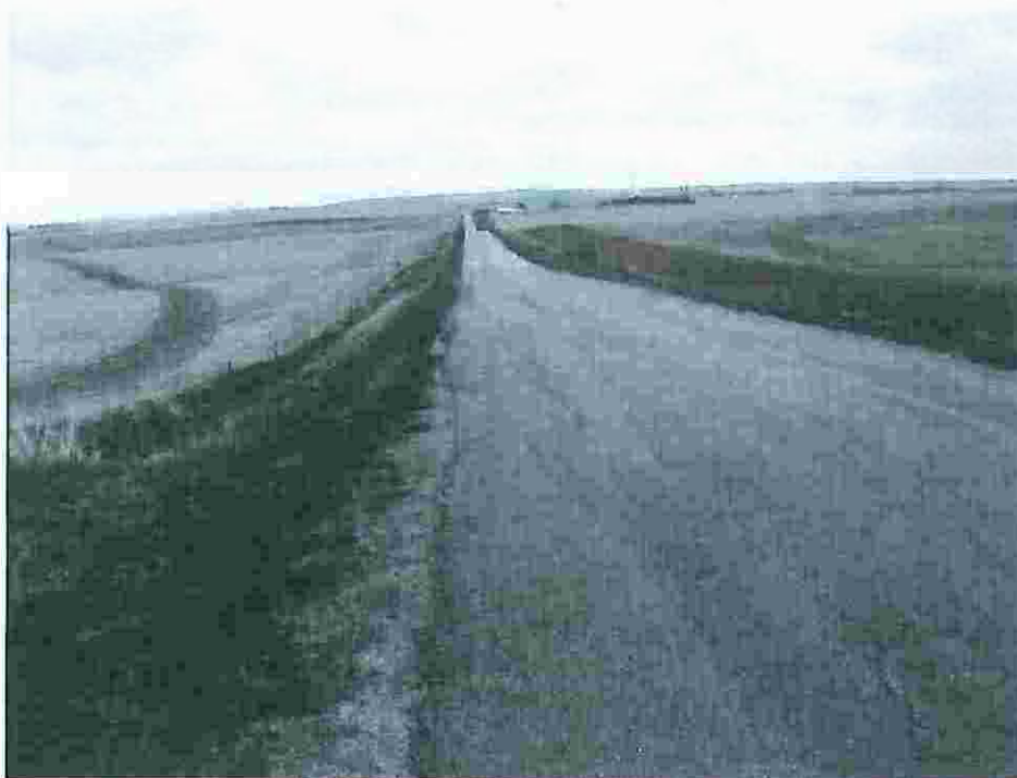
Photo #6236 1/4 mile line (north side of road) looking east.
