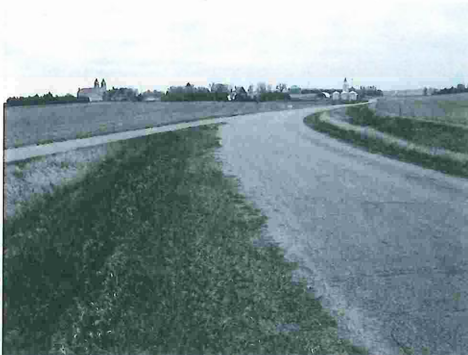
Photo #6245 1 ½ miles exiting curve, looking south-southeast.
