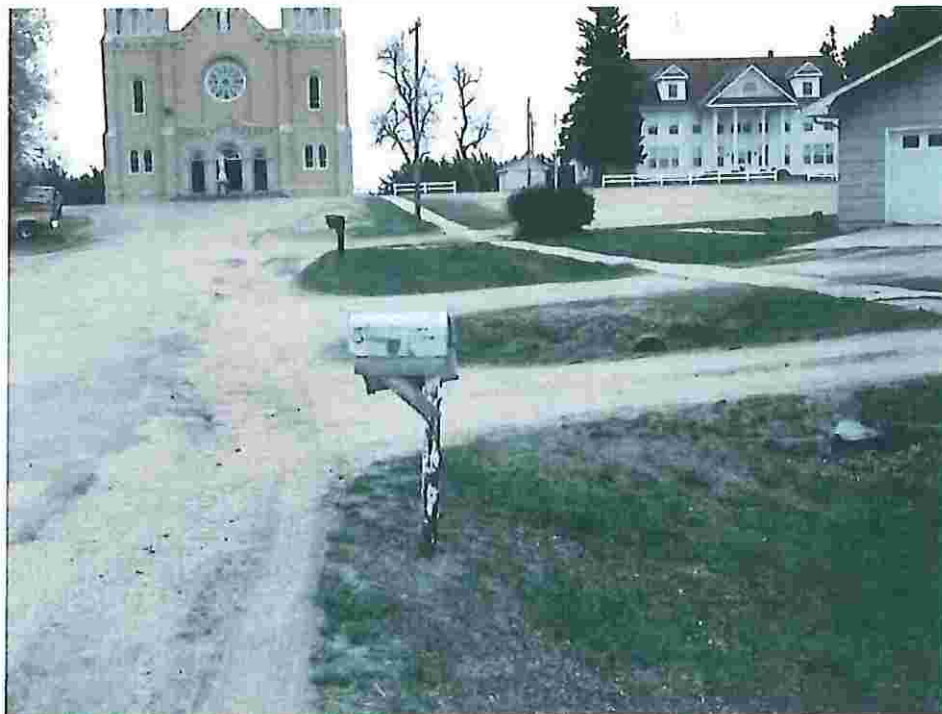
Photo #6252 Driveways looking east.
