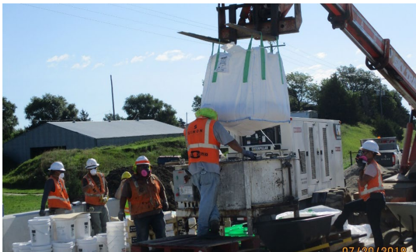
Figure 1.1 Proprietary UHPC batching during Belden-Laurel Bridge construction in 2018
