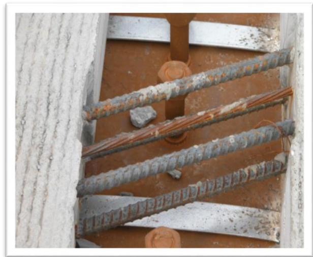
Figure 1.2: Threading post-tensioning strands (left) and conflicts between deck reinforcement and shear connectors (right)
