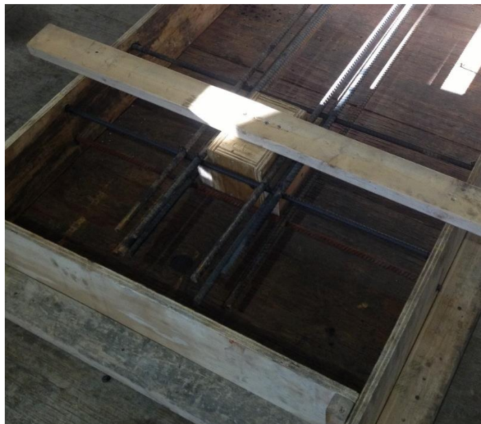
Figure 5.27: Wood-formed pocket with shear key
