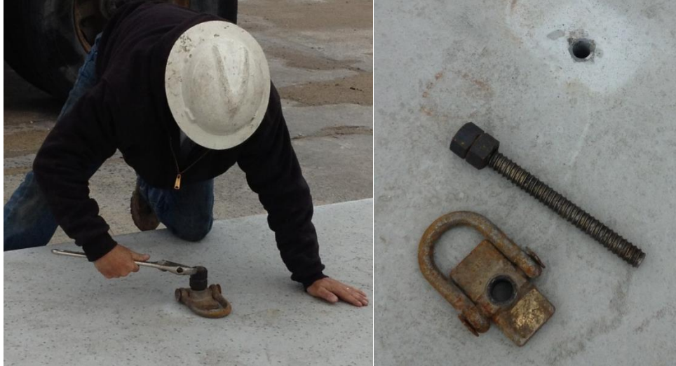
Figure 6.7: The coil rod with nuts and swivel plates used for panel lifting
