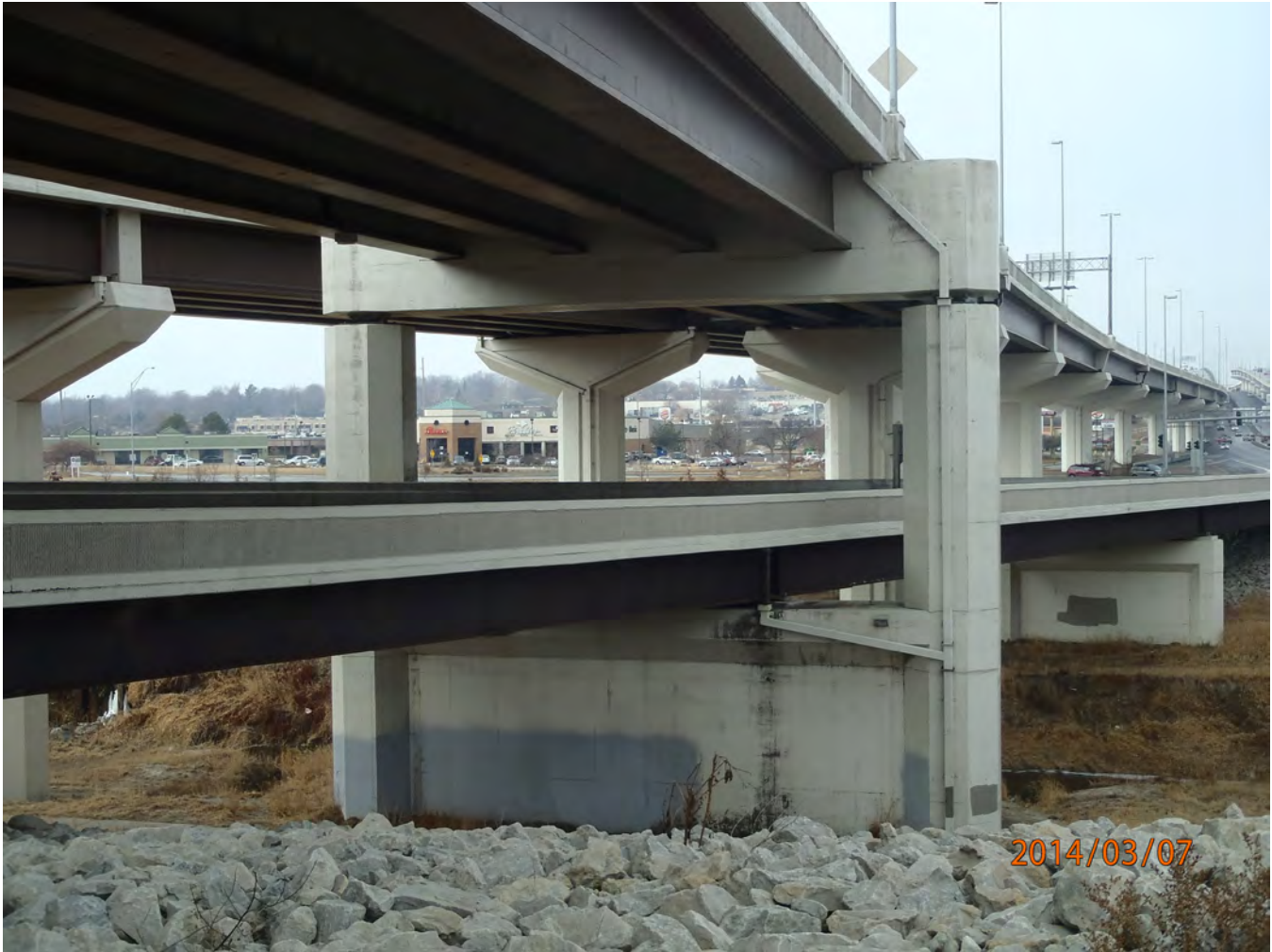
Structure N o : S006 36428A (upper) and S006 36466A (lower) The upper structure is classified as a straddle pier and the lower as a wall pier.
