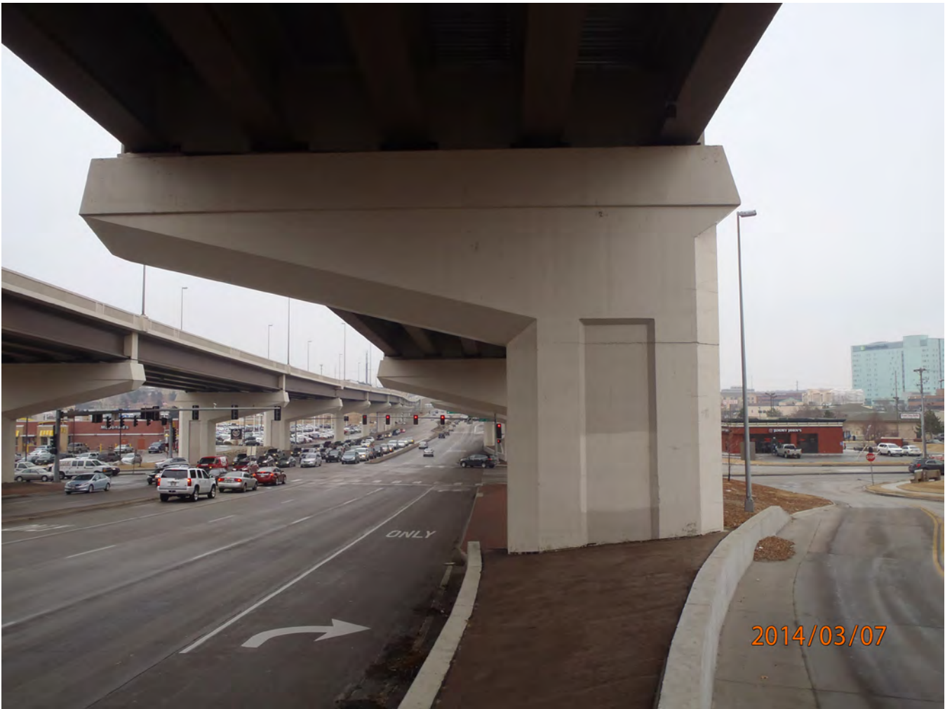
Structure №: S006 36428A
