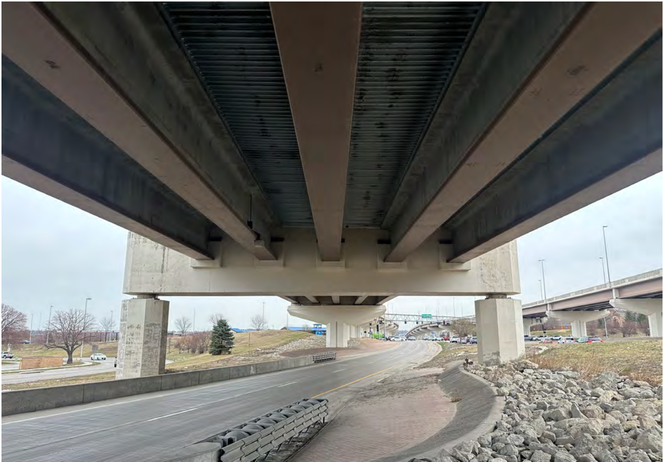
Structure Nº: S006 36428B
