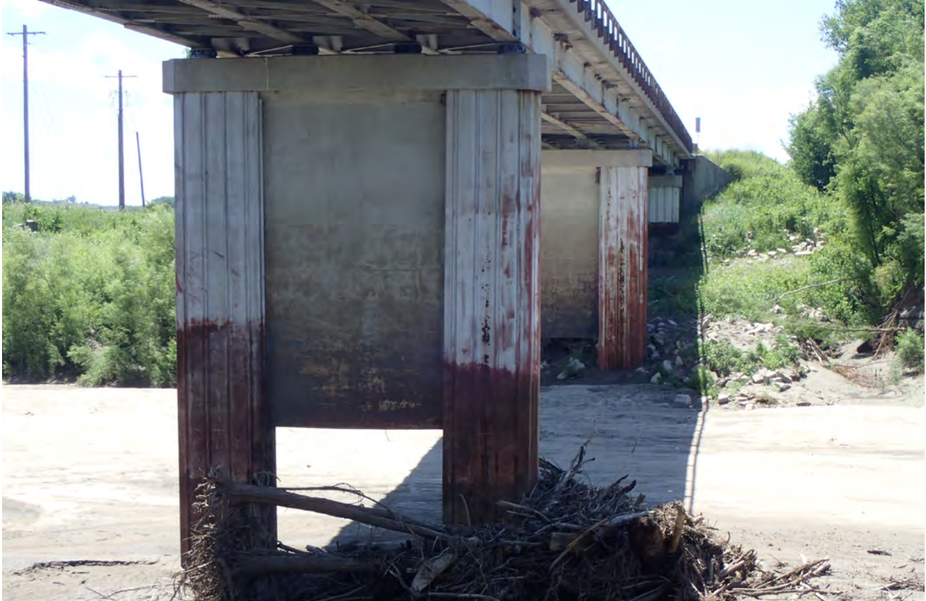
Structure No: S067 03943
