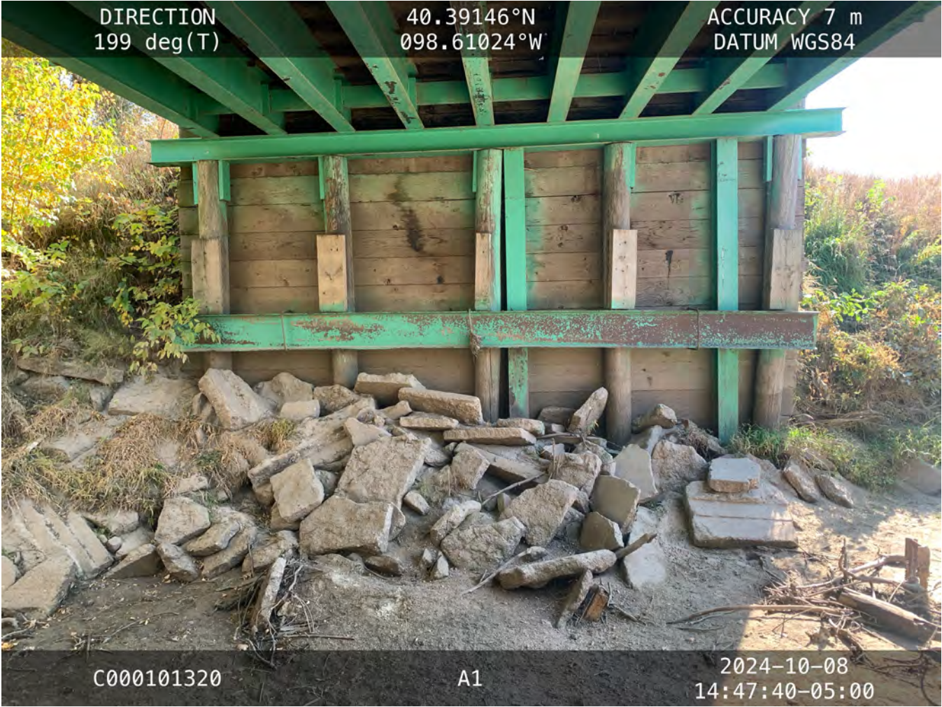
Structure Nº: C000101320
