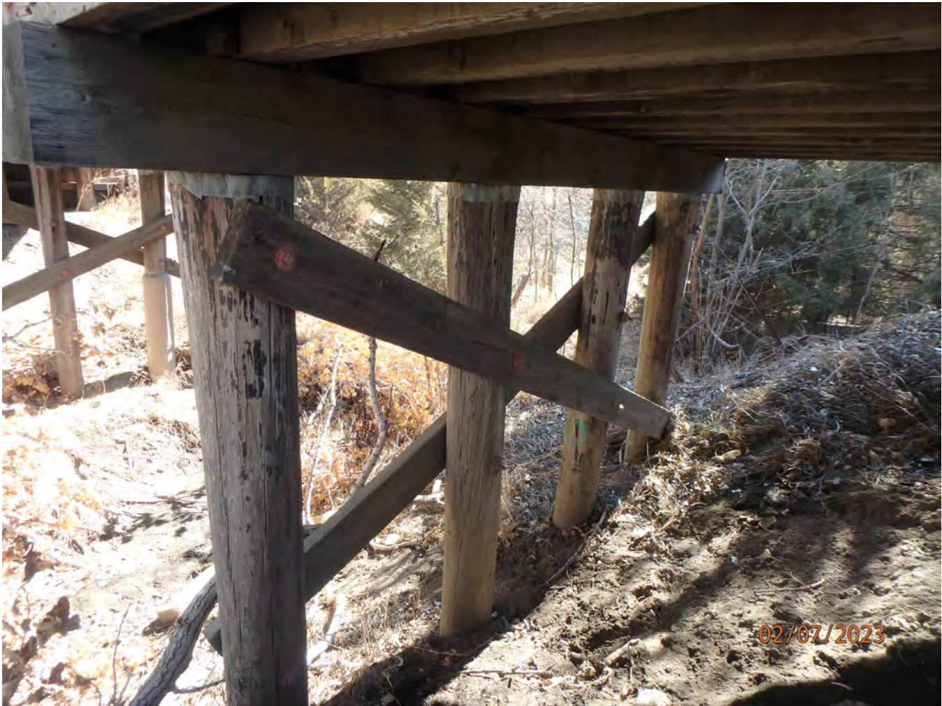
Structure №: S080 40872A
