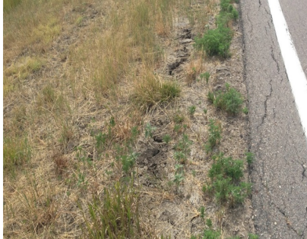
Figure 3.2 Longitude crack on top of the Verdigre slope at Highway 84 (Song et al., 2018)
