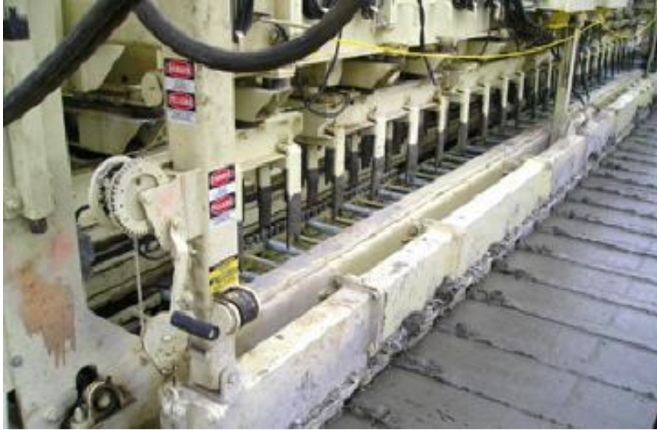
Figure 1.2 Dowel Bar Inserter (DBI)
