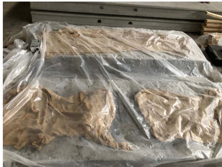
Figure 5-7. Curing of casted patches
