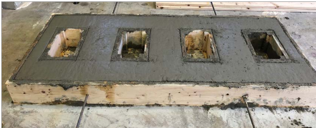
Figure 5-3. Concrete slab after casting
