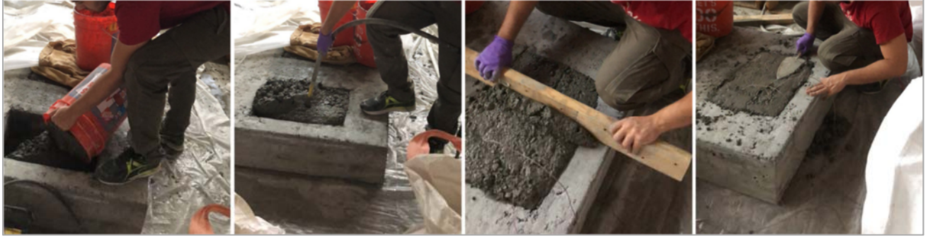
Figure 5-5. Slab patching process
