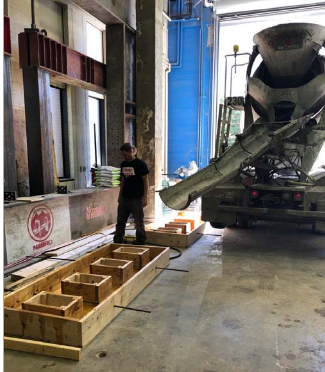
Figure 5-2. Concrete placement
