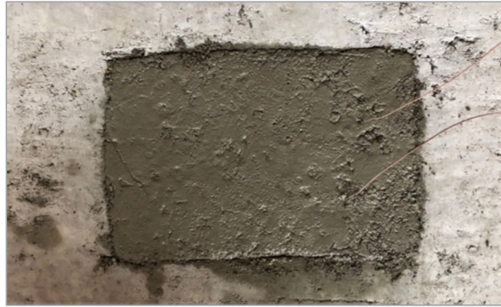
Figure 5-6. Finished patch surface
