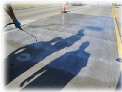
Figure 2. Sealer Application by Industrial Sprayer
