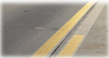
Figure 14. Panel Joints without Shading
