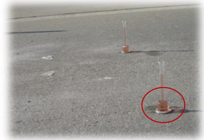
Figure 11. Measuring Fluid Leakage
