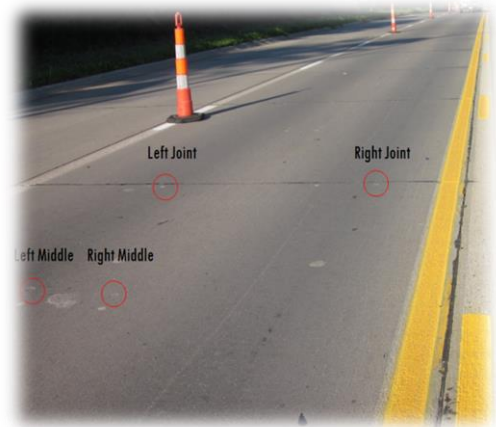
Figure 15. Chloride Ion Sample Locations on the Panel 2012-2014
