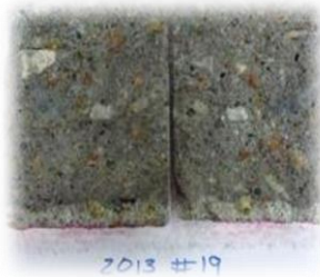
Sealer Penetration Visible
