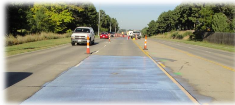
Figure 21. Sealer Dry Time After Application
