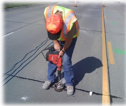
Figure 6. Chloride Ion Sample Drilling Inside joint, position (RT)
