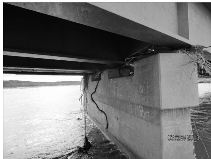
TYPICAL BEARING DEBRIS REMOVAL
