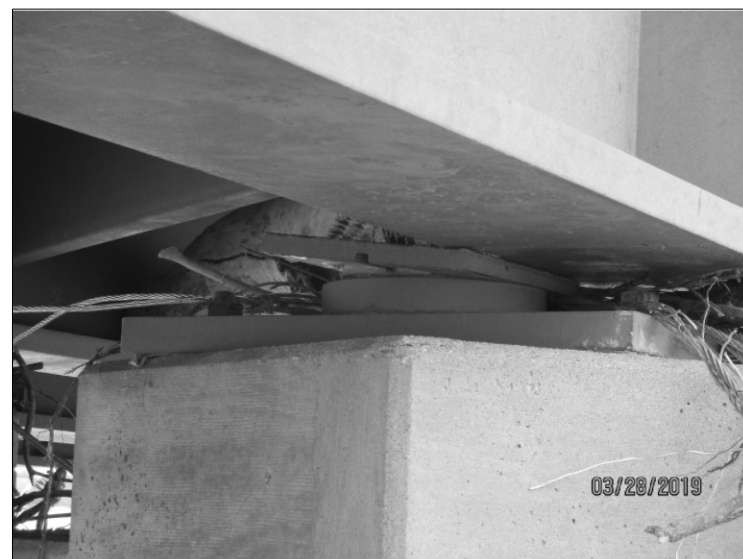
TYPICAL BEARING REMOVAL
