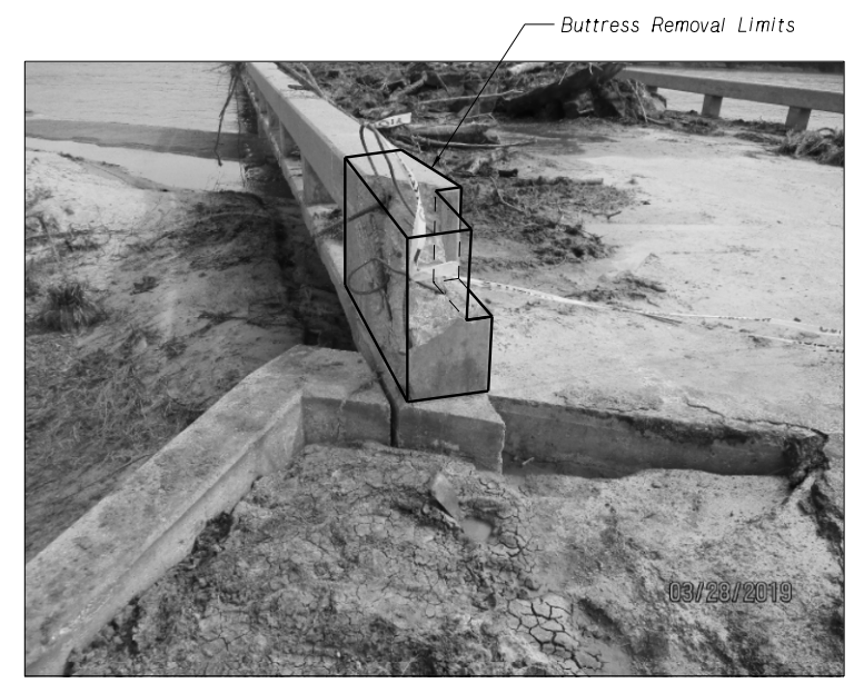
NORTHEAST BUTTRESS REMOVAL
