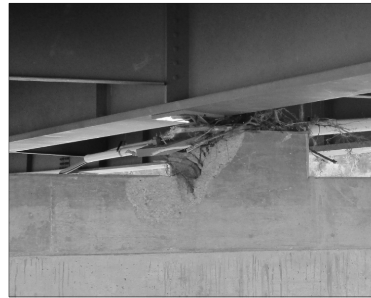
CONCRETE REPAIR - PIER NO. 5 NORTH FACE UNDER GIRDER B
