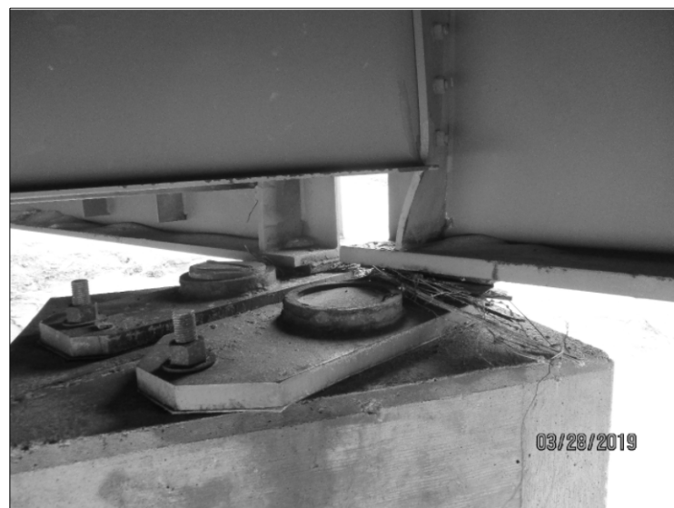
TYPICAL BEARING REMOVAL
