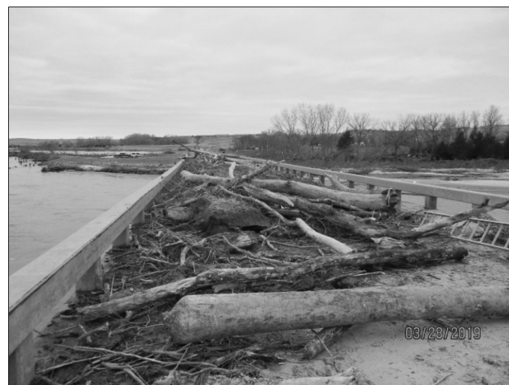
TYPICAL SUPERSTRUCTURE DEBRIS REMOVAL
