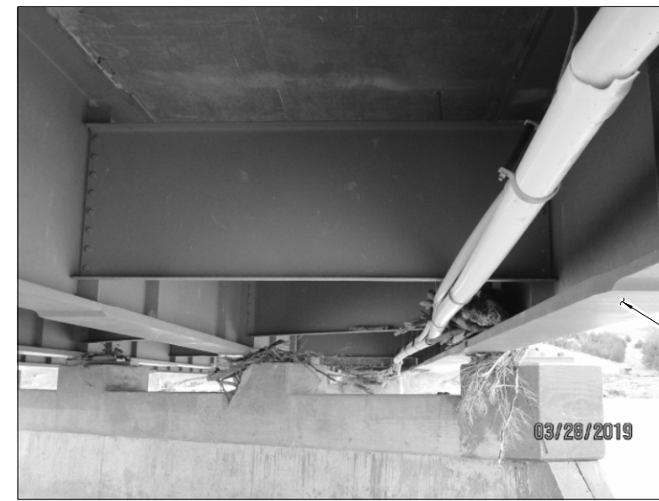
TYPICAL CONDUIT REMOVAL
