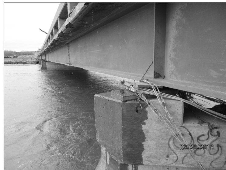
TYPICAL BEARING DEBRIS REMOVAL
