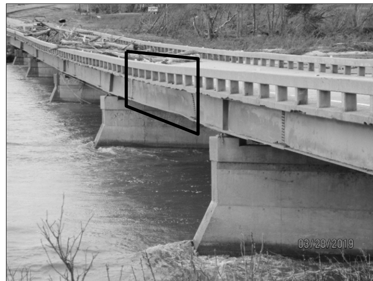
REMOVAL OF GIRDER A IN SPAN 3
