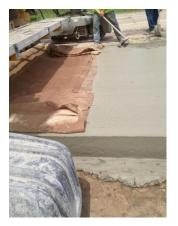
Figure 6. Placement of 40%RCA-60% 47B Fine
