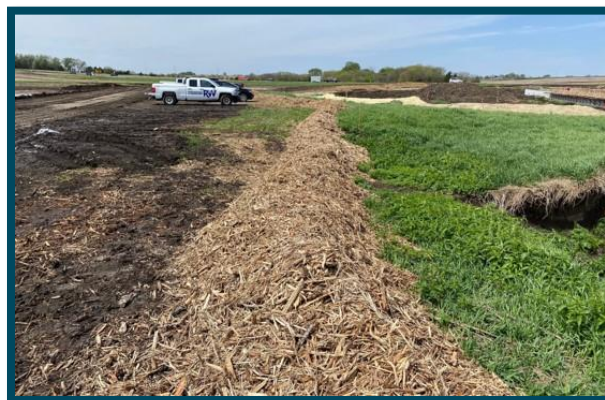
Figure 1: Slash mulch berms work well as perimeter control as a secondary BMP to existing grass buffer or cover crop.
