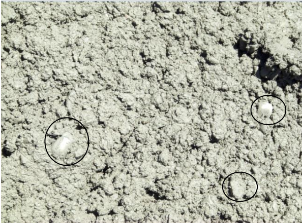
Figure 10. Aggregate's dust coating observed during paving operations.
