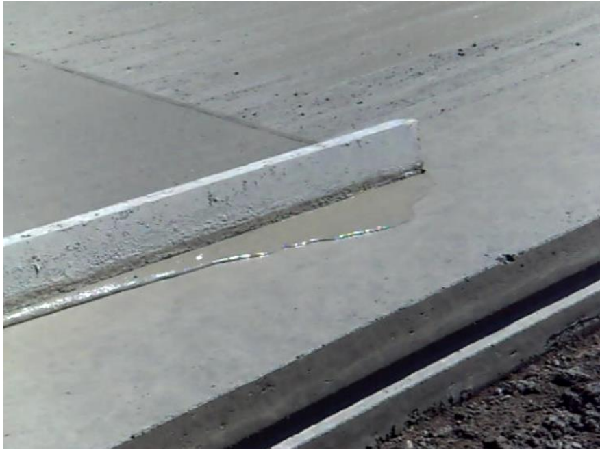
Figure 6. Slab Surface Tempered During Paving Operations.
