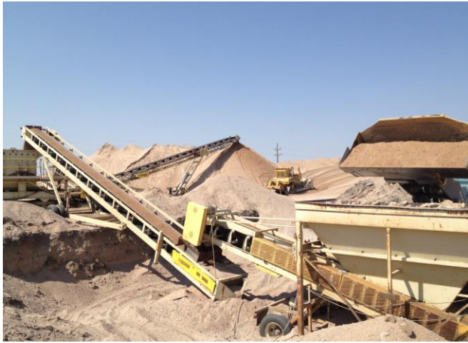
Figure 20. Aggregate Plant Site
