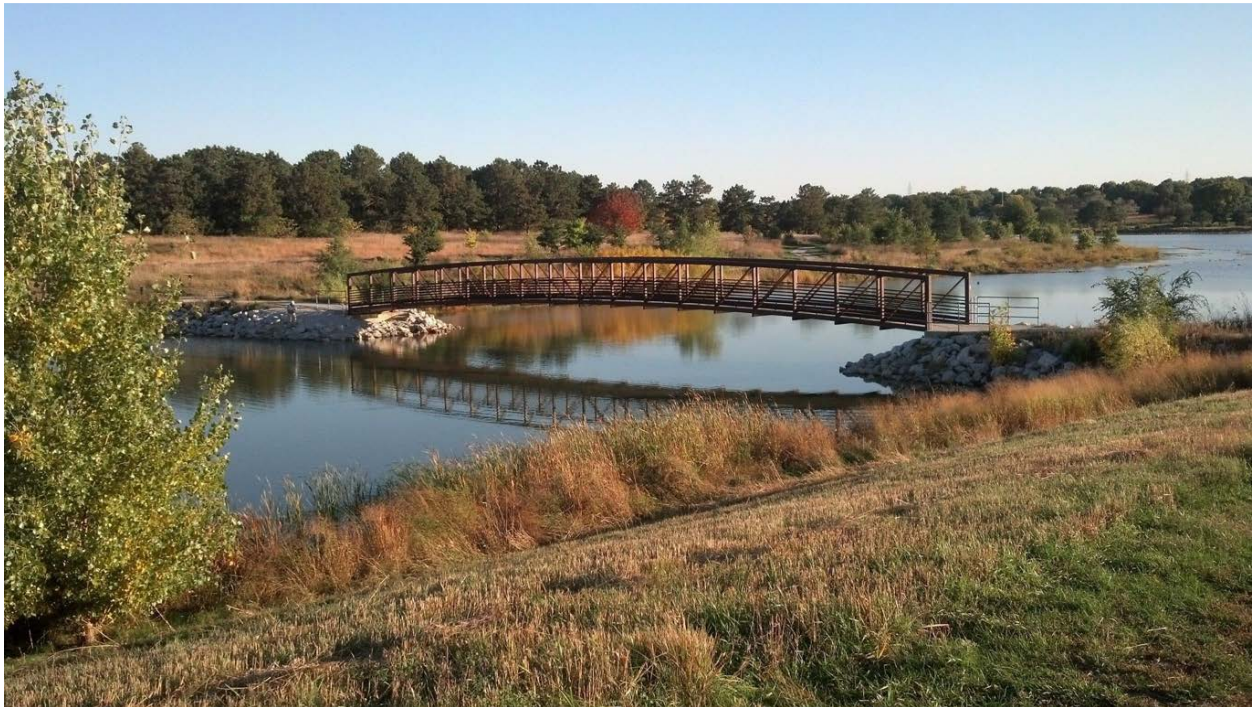
Figure 63: Holmes Lake footbridge.
