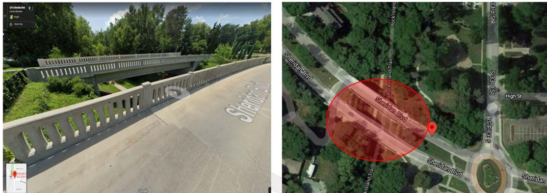
Figure 32: Street and satellite view of Sheridan Blvd. Bridge from Google Maps [23]
