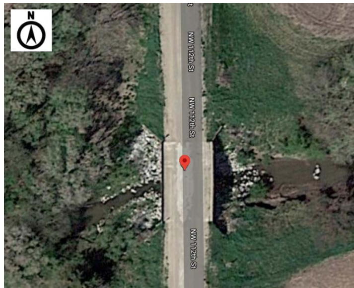
Figure 25: Satellite view of M-164 bridge from Google Maps (Geographical location: 40°49'20.4"N 96°52'22.7"W)
