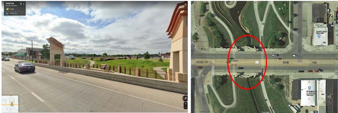
Figure 40: Street and satellite Views of O St. bridge from Google Maps [23].
