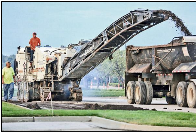
Asphalt Pavement Milling
