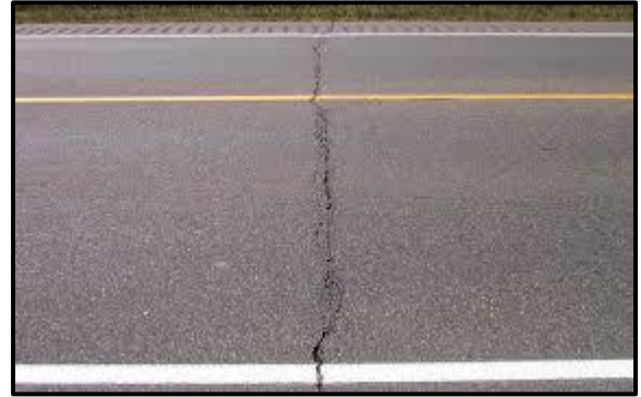
Transverse Cracking
