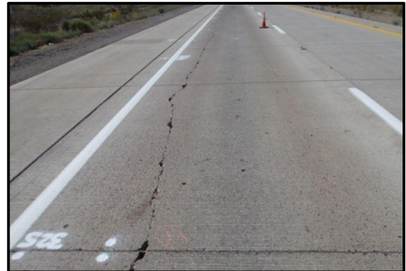
Slab Cracking
