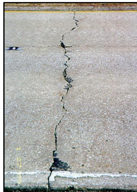
Transverse Cracking
