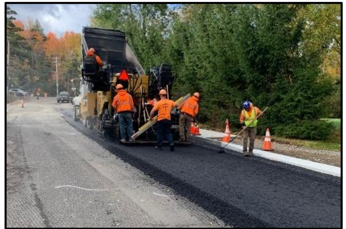
Asphalt Overlay Paving
