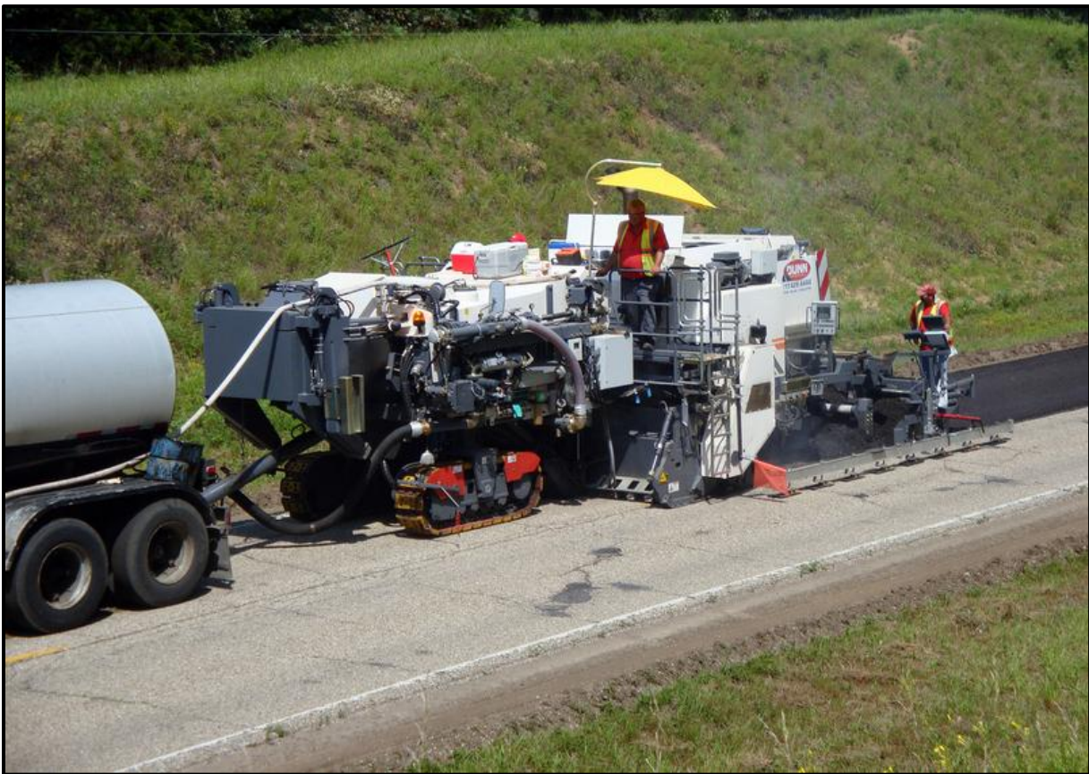
Cold In-Place Recycling
