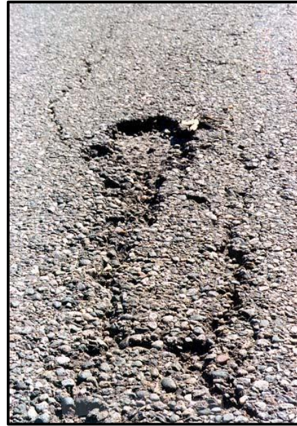
Raveling/Weathering
