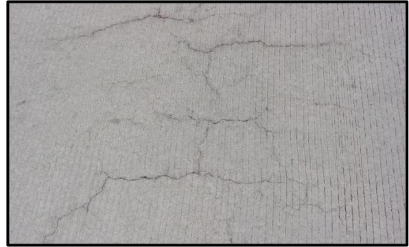
Pattern Cracking
