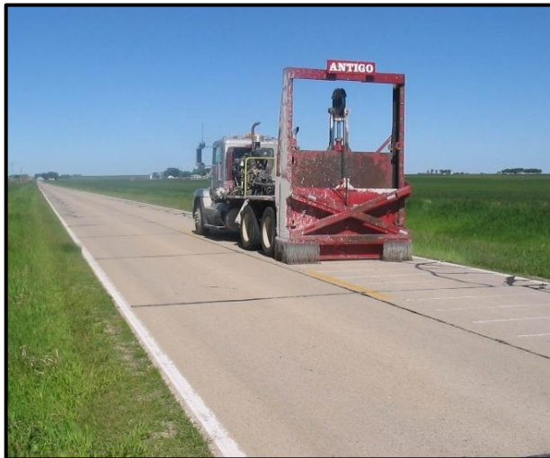
Cracking Concrete Panels
