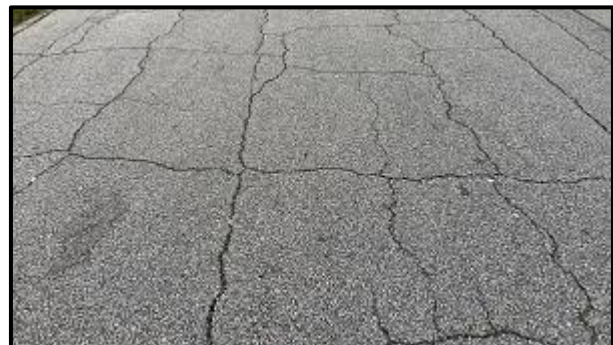
Block Cracking
