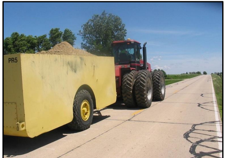
Seating Concrete Panels
