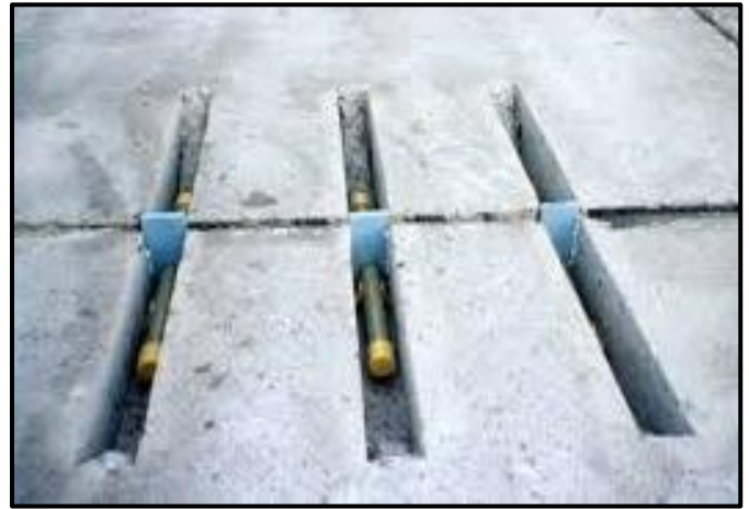
Dowel Bars Used in Dowel Bar Retrofit
