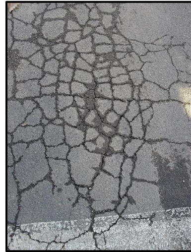
Alligator Cracking
