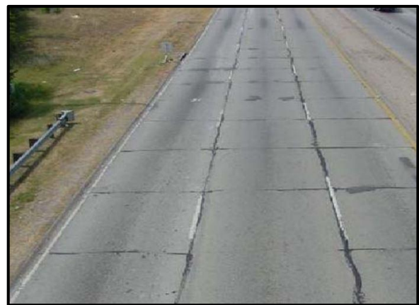
Reflective Cracking
