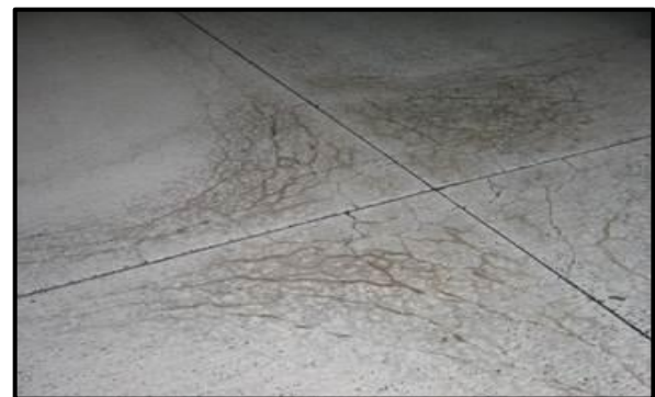
D-Cracking
