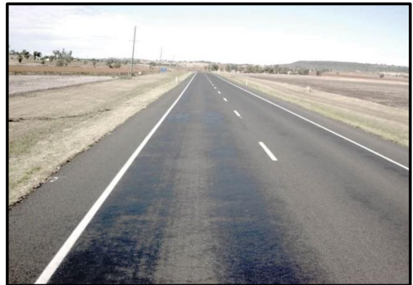
Bleeding/Flushing
