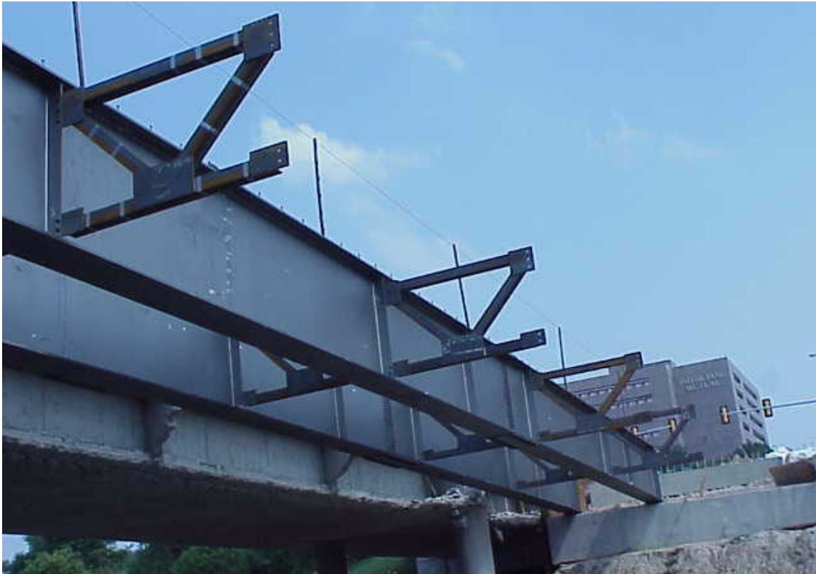
Figure 3-11: Girder sections 4 and 5 of the East span
