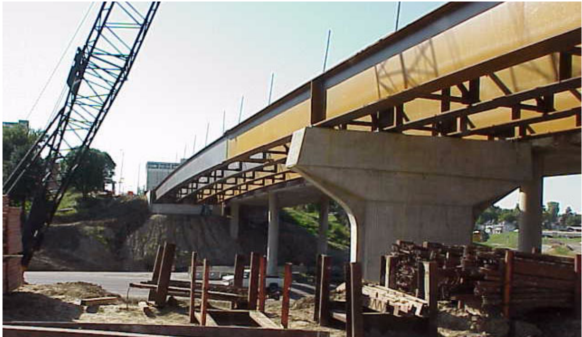
Figure 3-13: West span girders in place
