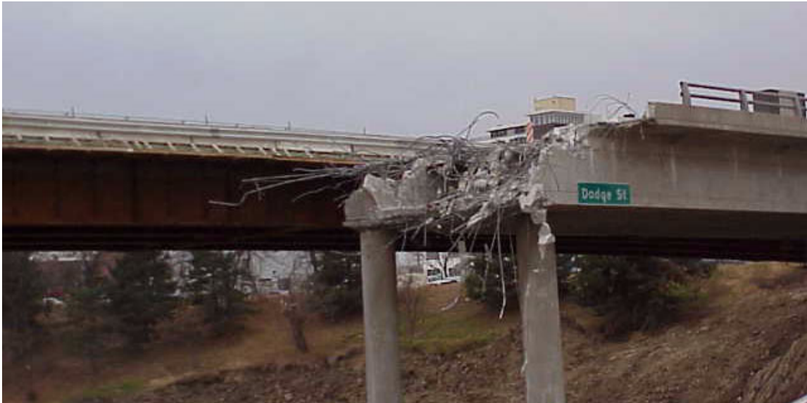
Figure 3-18: Demolition of the Northern half of the existing bridge
