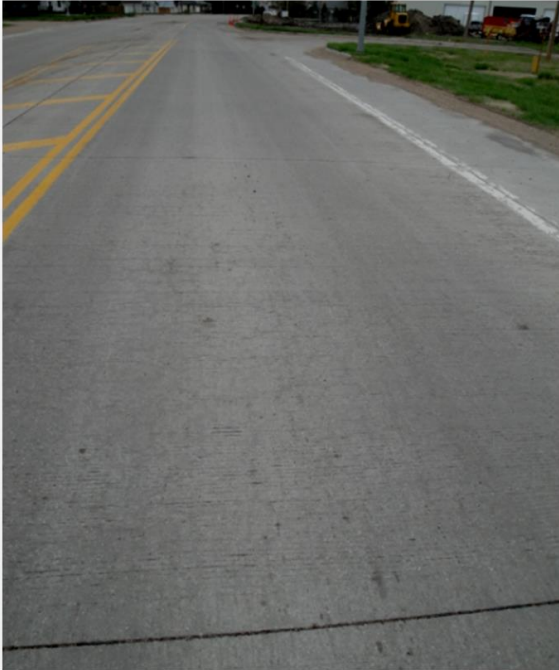
Figure 6 - Field Performance (Highly Reactive Aggregate) Ansley built 2001
