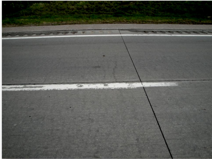
Figure 9 - Field Performance (Very Highly Reactive Aggregate) Norfolk East built 2004
