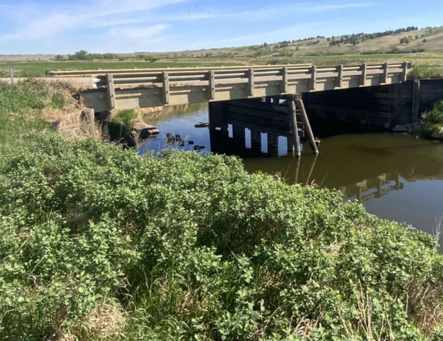
Split, Pile 3 and 4 of the east abutment, only bearing approximately 20%
