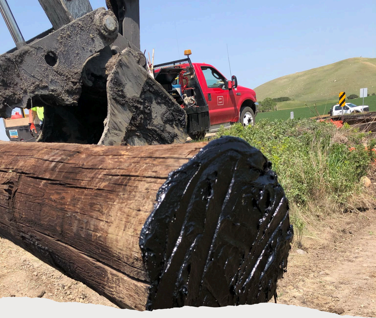
Rotted Piling Repair
