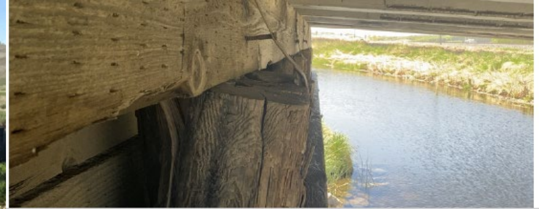
Split, Pile 3 and 4 of the east abutment, only bearing approximately 20%
