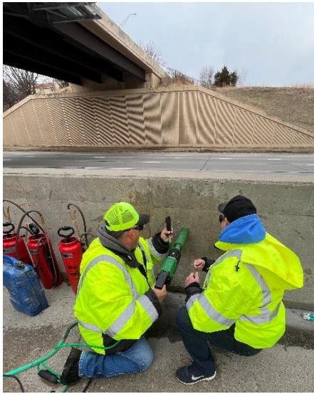
Figure 2 - The coring crew used a handheld coring drill to cut cores from the barrier.
