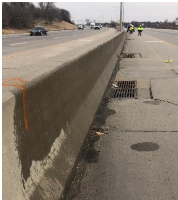
Figure 7 - The power washed section after sealer was applied.
