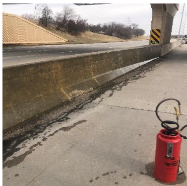
Figure 4 - PCS was applied to the designated control section.
