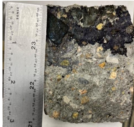
Figure 8 - The power washed section core before sealer was applied.
