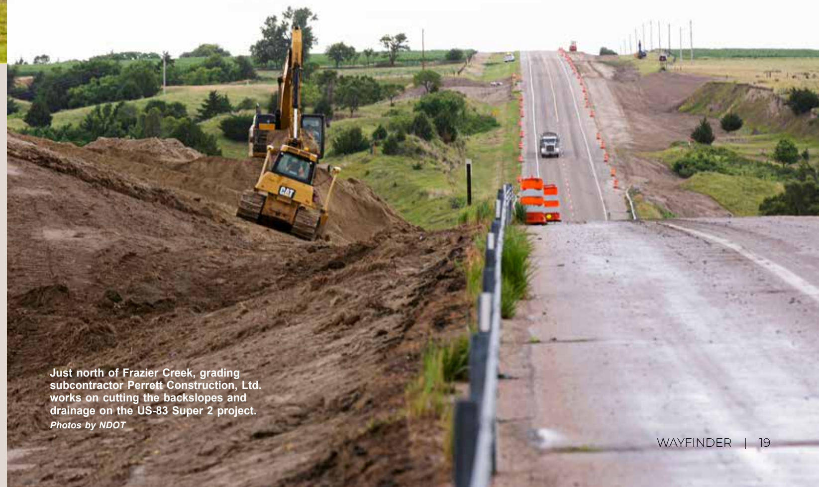
Grading subcontractor Perrett Construction, Ltd. hauls dirt from excavation sections to fill sections on the US-83 Super 2 project, "Frazier Creek North and South."
