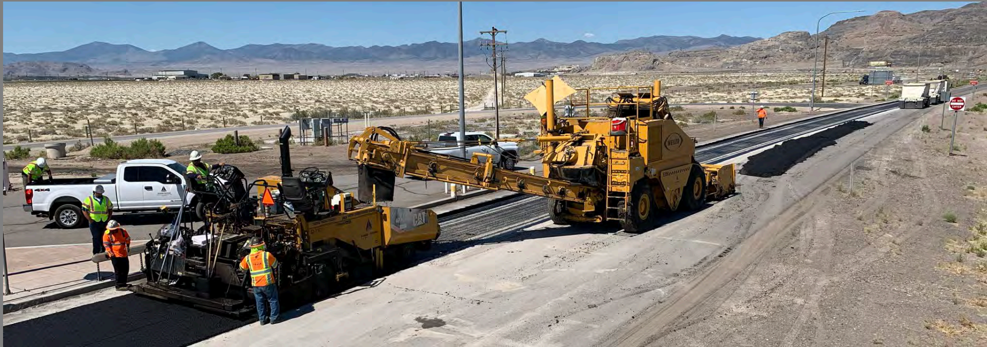
I-80 East Bound Port of Entry Ramp June 3, 2021
