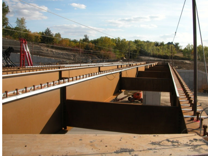
Figure 36 Support System in Skyline Bridge.
