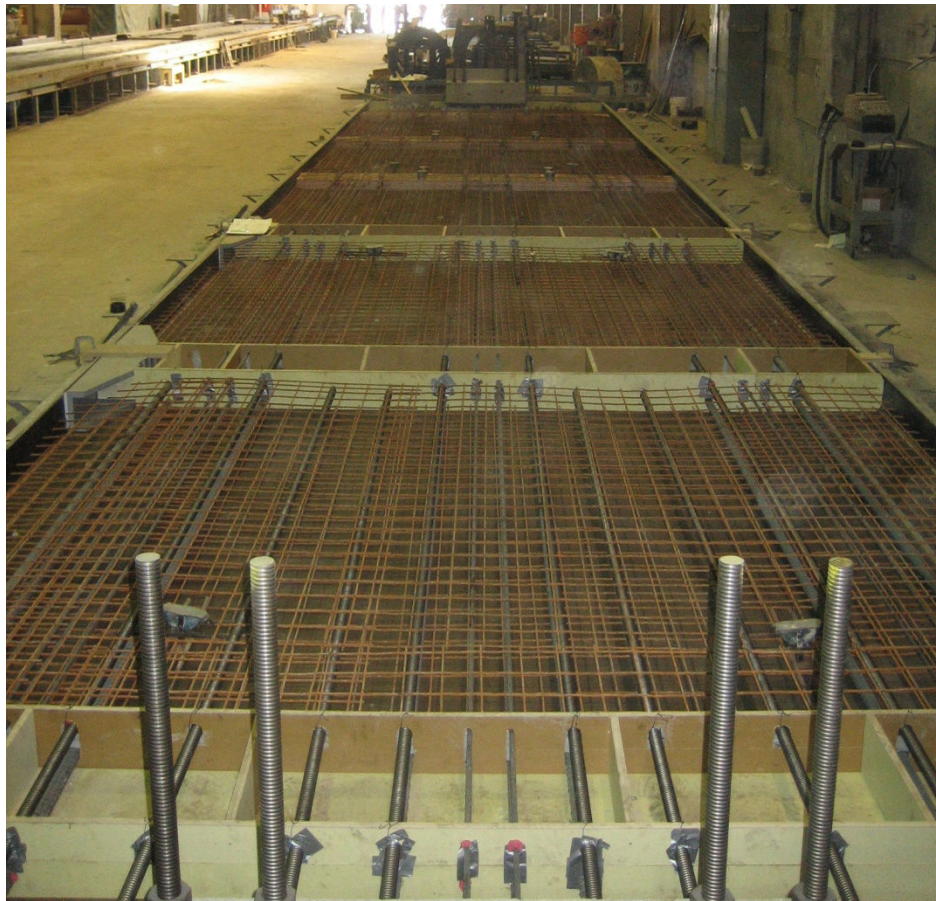
Figure 67 Demonstration panel reinforcement setup and formwork.
