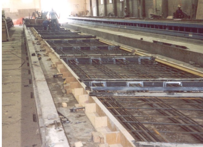
Figure 24 Reinforcement Setup of Skyline Bridge Panel.
