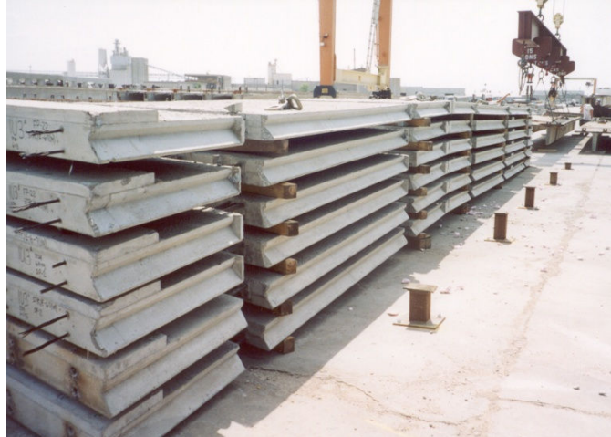
Figure 30 Crown Panels Stacked Up in the Precast Yard.
