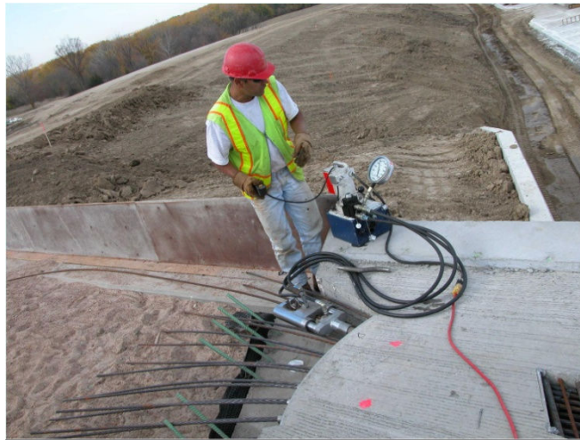
Figure 49 Post-tensioning Strands.
