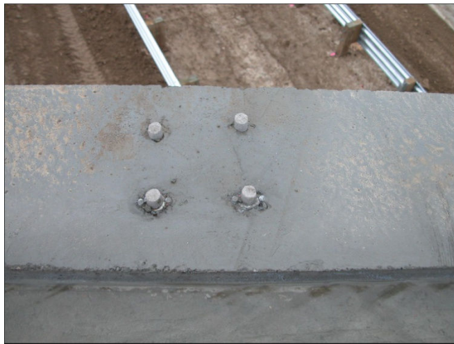
Figure 55 Galvanized Female Insert.
