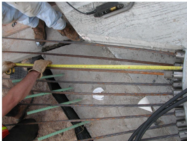
Figure 50 Measuring Strand Elongation.
