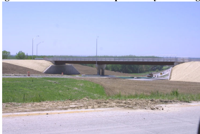
Figure 59 Elevation of Completed Skyline Bridge.
