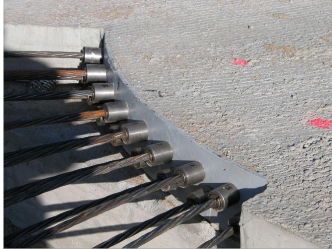
Figure 48 Strands Anchored with Chucks.
