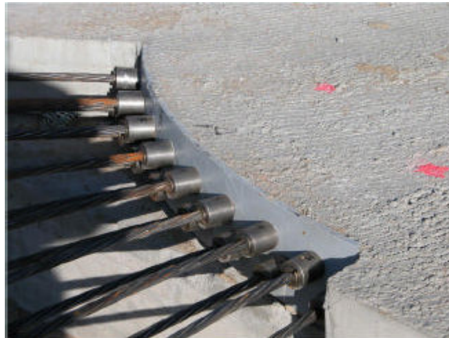
Figure 19 Special anchorage device in end panel of Skyline Bridge.
