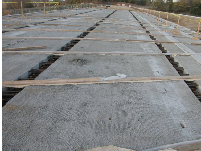
Figure 45 Curing the Shear Key.
