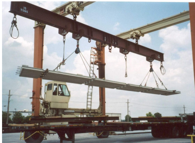
Figure 28 Skyline Bridge Panel Handling.
