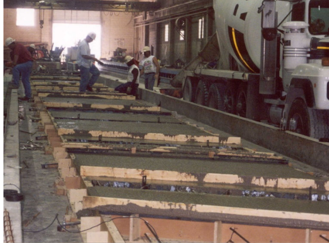
Figure 27 Pouring the Precast Deck.
