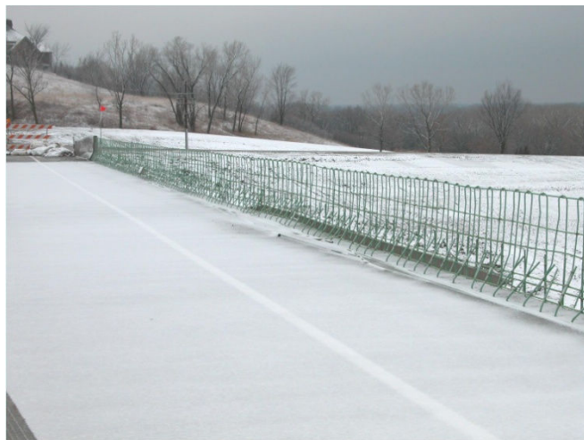
Figure 56 Barrier Reinforcement.
