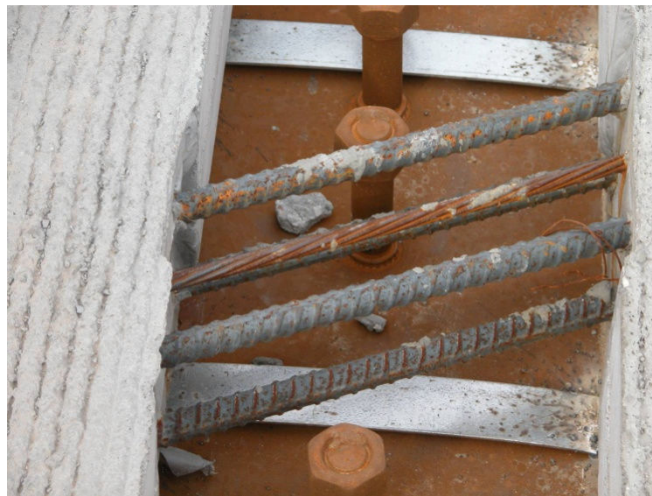
Figure 43 Channel Details before the Post-tensioning Strands are Pulled Through.
