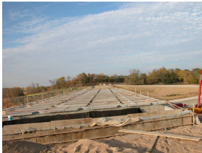
Figure 46 Plan View of Skyline Bridge before Post-tensioning.
