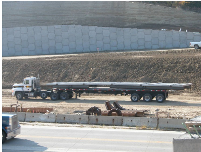
Figure 33 Skyline Bridge Panel Shipping.
