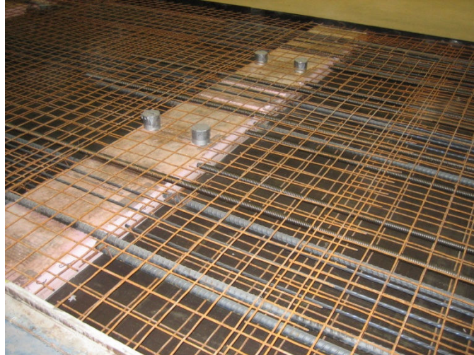
Figure 71 Girder line with mid-depth duct and vent tubes.
