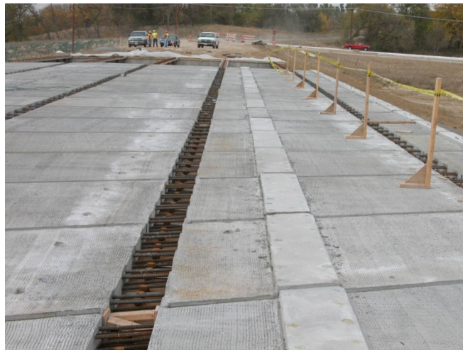
Figure 41 Another Plan View of Skyline Bridge Panels.
