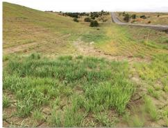
Pictured far left: Earth checks should be used in conjunction with other BMPs such as perimeter controls. Checks used adjacent to wetlands, waterways and sensitive areas shall include secondary BMP to prevent the discharge of the check material.
