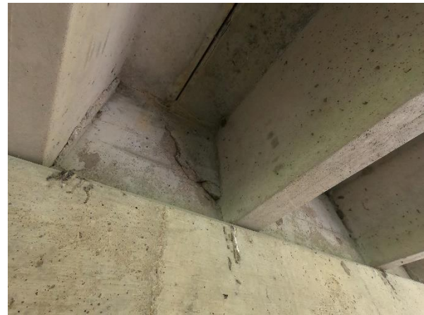
Figure 4: Cracks in X084, recorded in 2024
