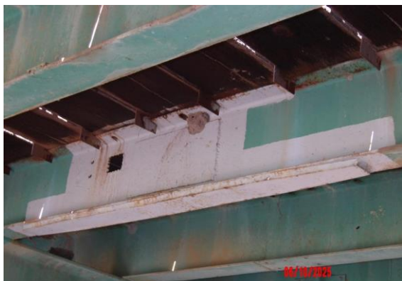
Figure 7: Repair on Stringer
