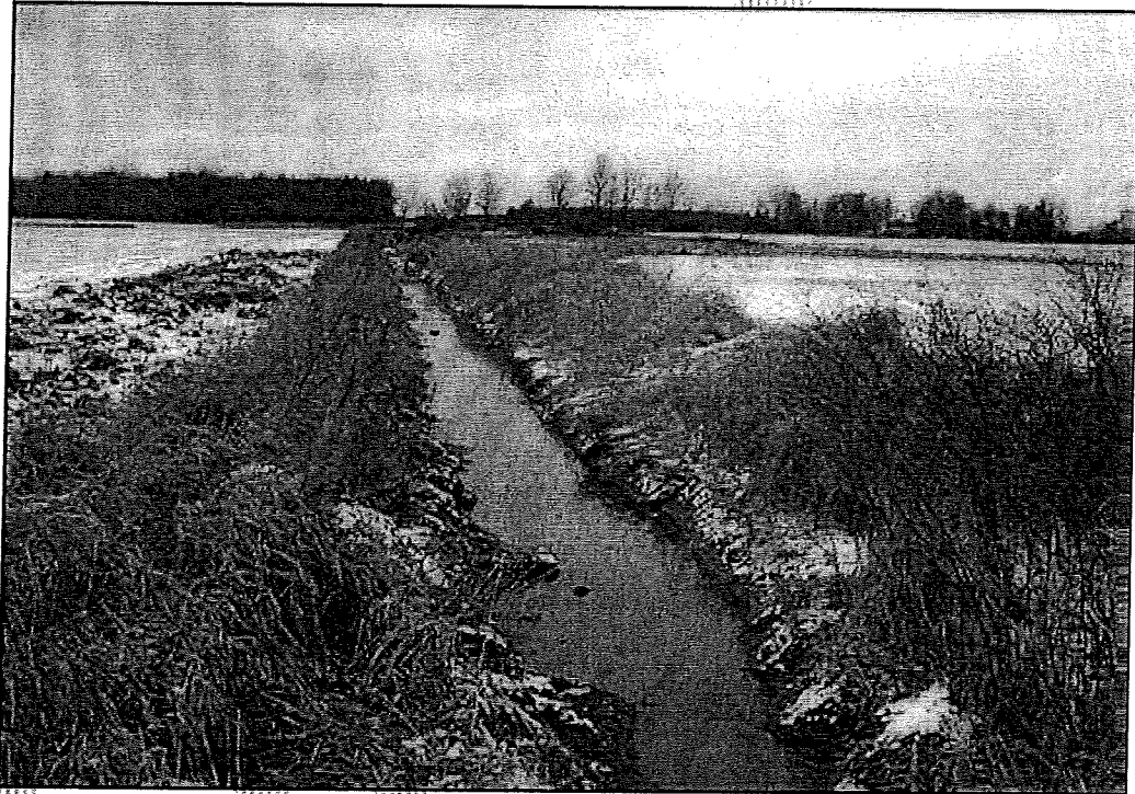
Figure 2.2 A typical modified headwater stream in Midwestern United States (Ward et al. 2008).
