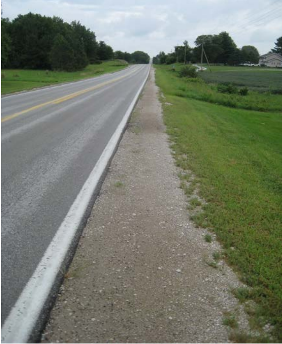
Figure 5 – Concrete Millings Incorporated into Shoulder on NE 66.
