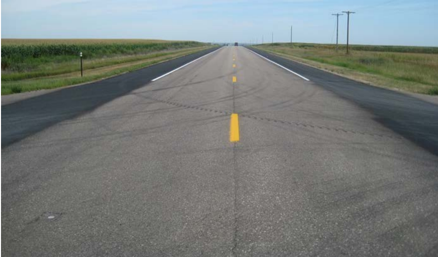
Figure 7 – Paved shoulders on NE 61 South of Ogallala.
