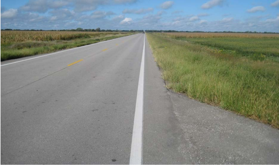
Figure 6 – 12-Foot-Wide Lanes on 14-Foot-Wide Pavement (NE 41 west of Wilber).
