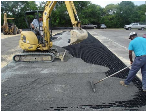
Figure 20 – Constructing Parking with Geopave.
