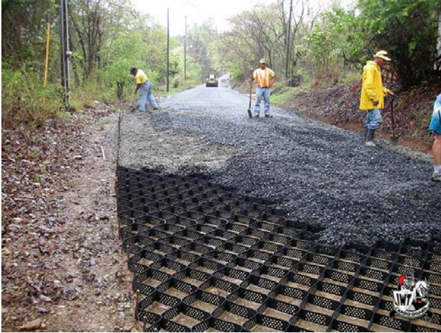
Figure 18 – Envirogrid Used as a Road Base.
