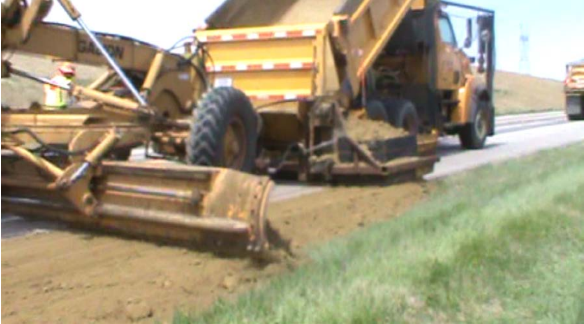
Figure 4 - NDOR District Maintenance Crews Adding Soil to Shoulder.
