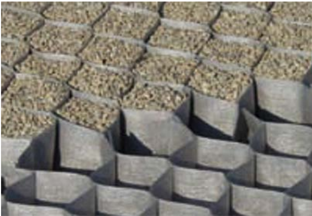
Figure 17 – Stabilization Grid Partially Filled.
