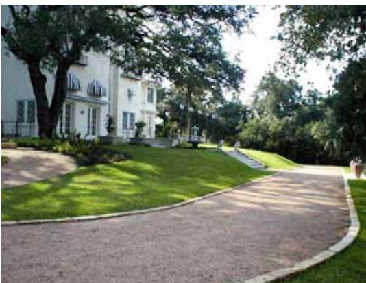
Figure 19 – Driveway Constructed With Gravelpave2.
