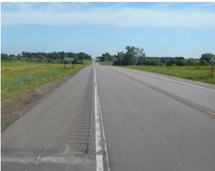
Figure 8 – Rumble Strips on Shoulder (US 77 South of Beatrice).
