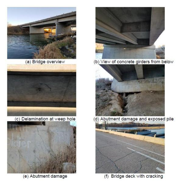
Figure C.1. Sample images of the concrete girder bridge.
