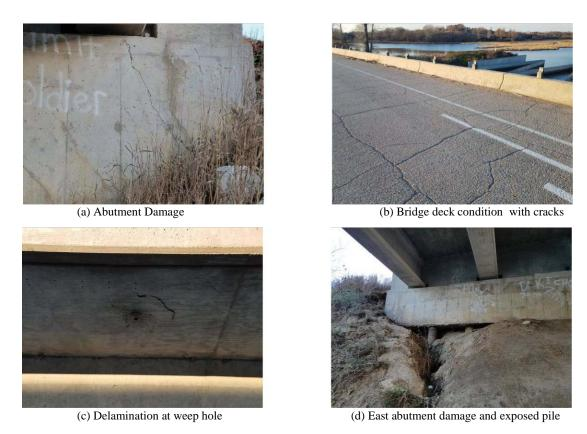
Figure 2.7. Damage example images of the NOBL North bridge in Omaha site.
