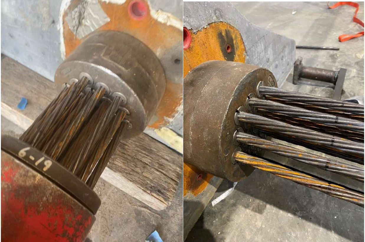
Figure 5.39: Anchorage plates and the hardware used for post-tensioning.
