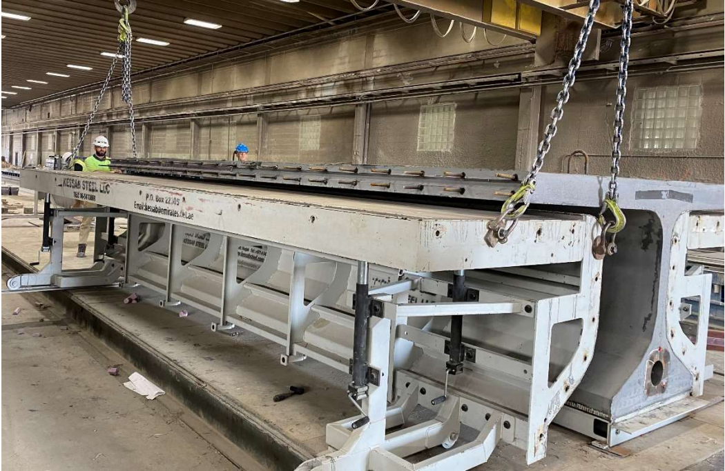
Figure 4.26: Stripping side forms of DIB with solid slab
