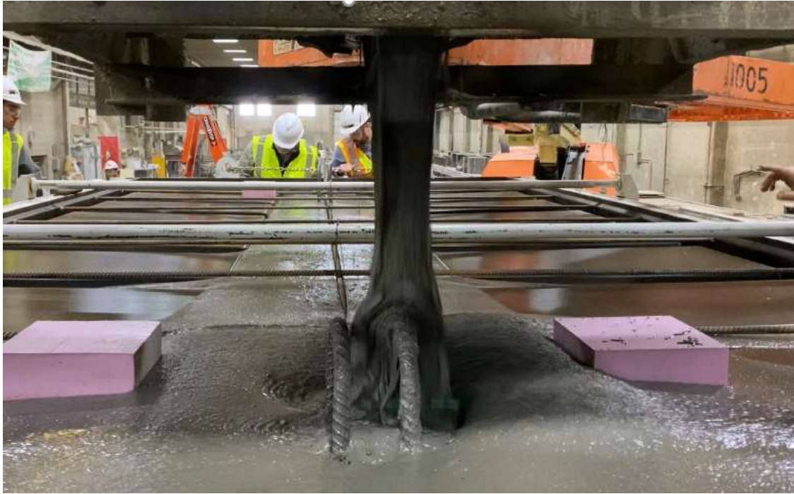
Figure 4.15: Casting UHPC from one end using bucket
