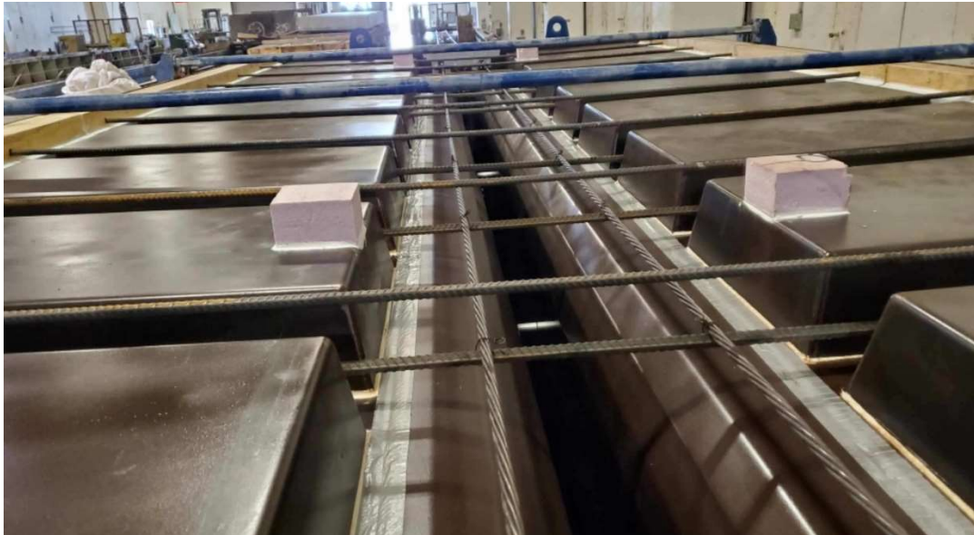
Figure 4.3: Forms and reinforcement of UHPC pretensioned specimen
