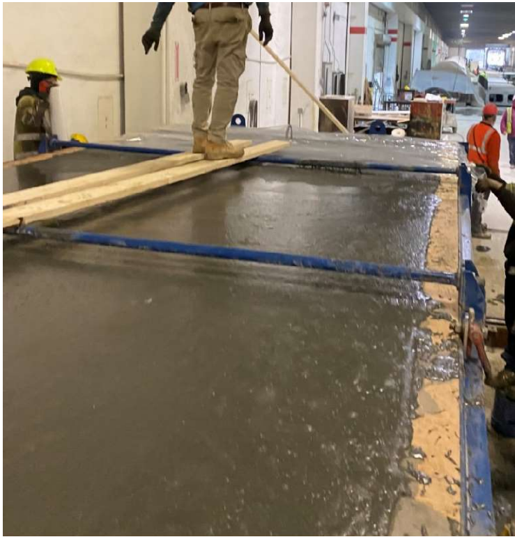
Figure 4.6: Finishing UHPC top surface and covering with plastic sheets
