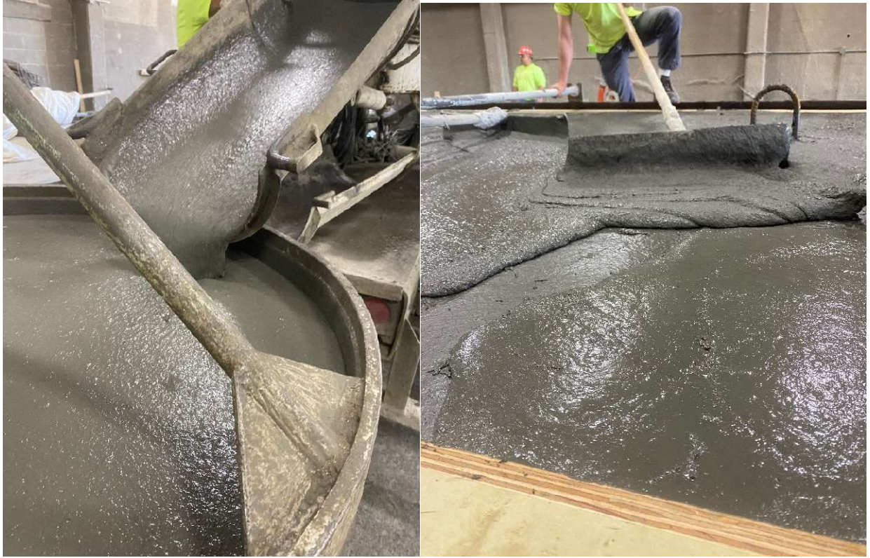
Figure 4.24: UHPC flowability during casting
