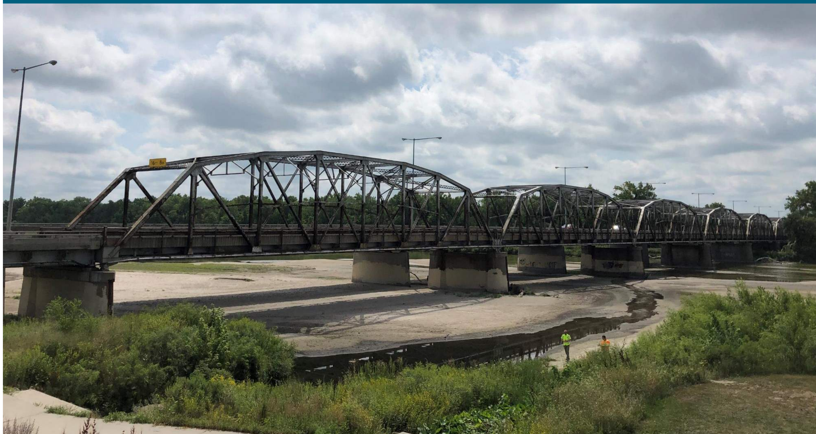
S030 37773L: Southbound Bridge
