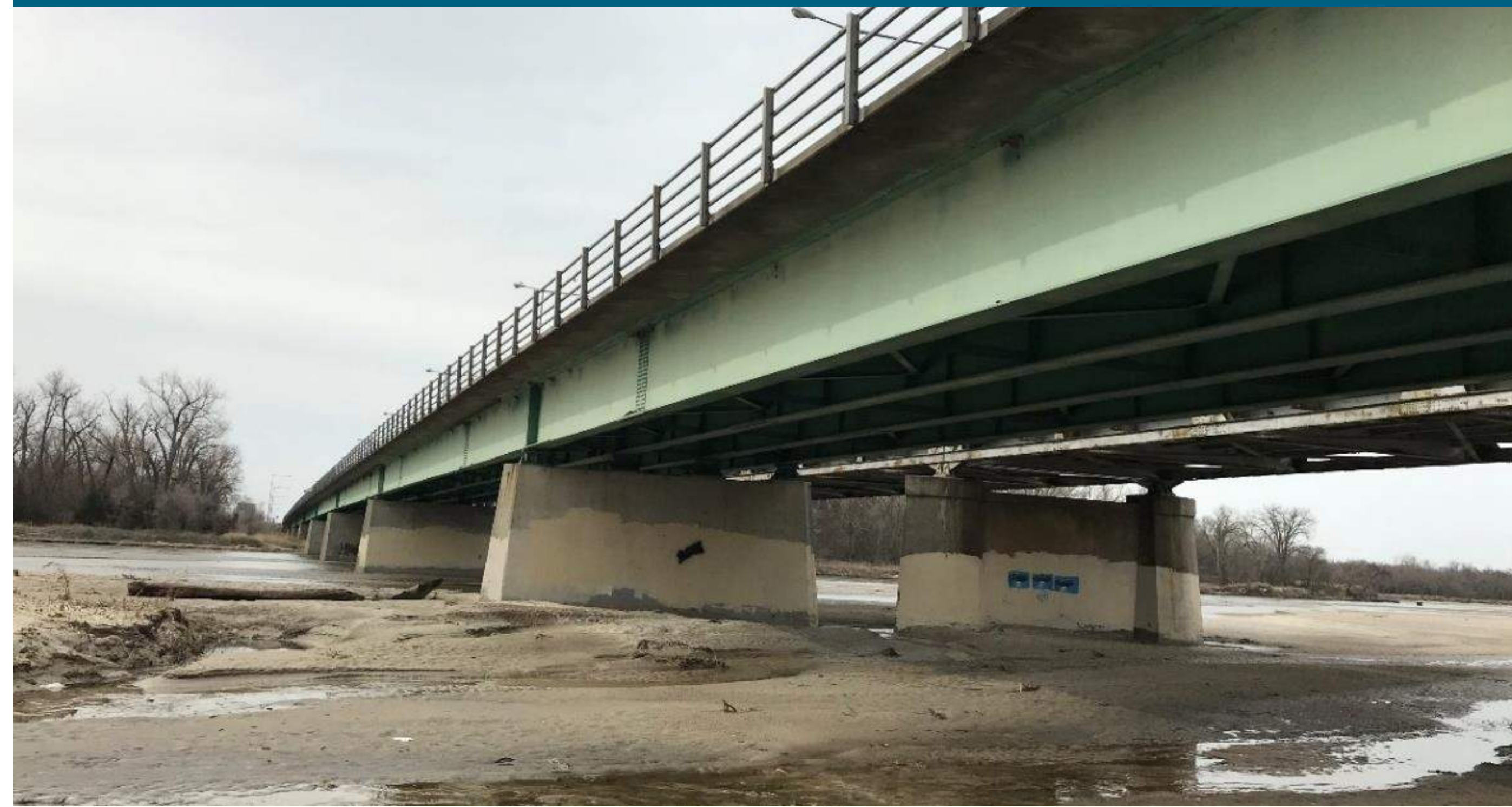
S030 37773R: Northbound Bridge
