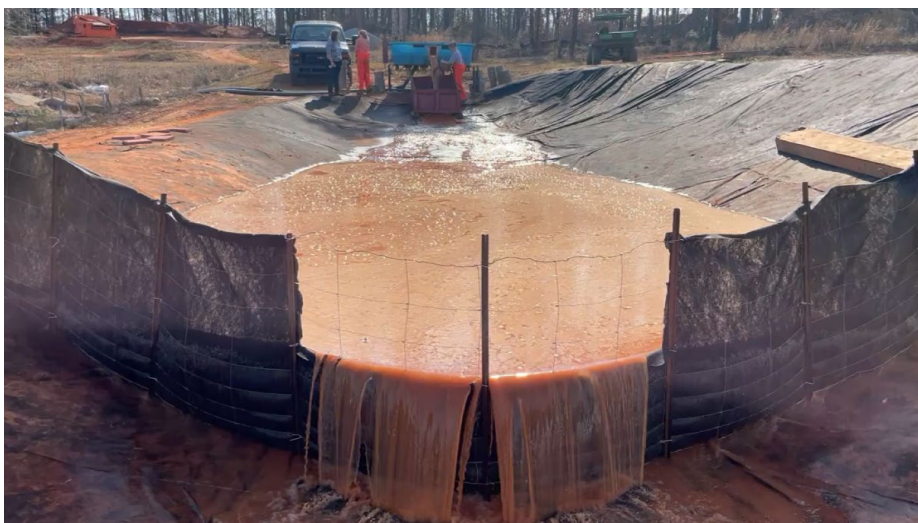
Figure 1: Modified silt fence design (nonwoven, wire backed, 18" weir, V-shape in channel).
