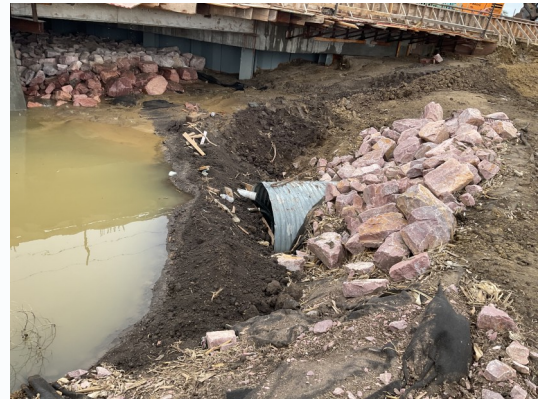
Blocking the flow of water at a temporary channel crossing would be an Immediate Corrective Action on a project
