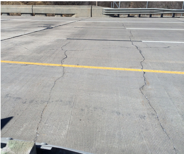
C. Good candidate for cross-stitch repair (photo taken from S080 42697L)
