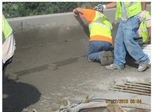
Figure 7.33—Concrete Patching at Bridge Rail, with Shotcrete
