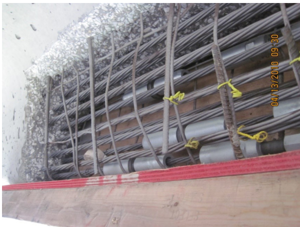
E. Splices Installed
