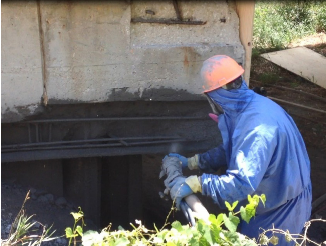
Figure 7.31—Concrete Patching at Abutment with Shotcrete
