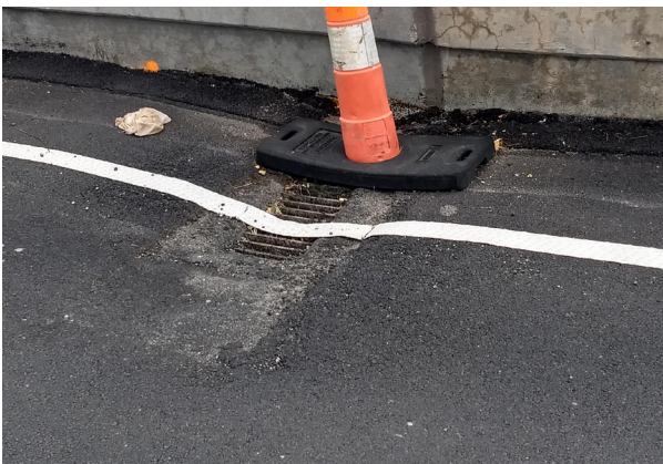
Figure 7.47—Drain in Driving Lane
