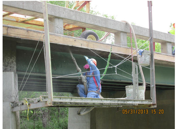
Figure 7.32—Concrete Patching at Deck Edges, with Shotcrete
