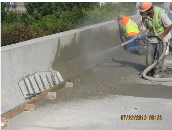
Figure 7.33—Concrete Patching at Bridge Rail, with Shotcrete
