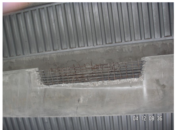
B. Concrete Removal
