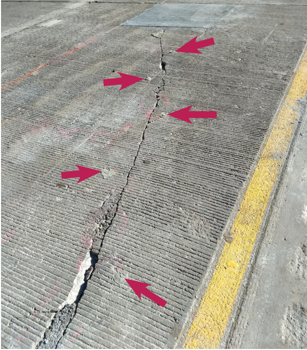
A. Completed cross-stitch repair (photo taken near SL28B00163L)
