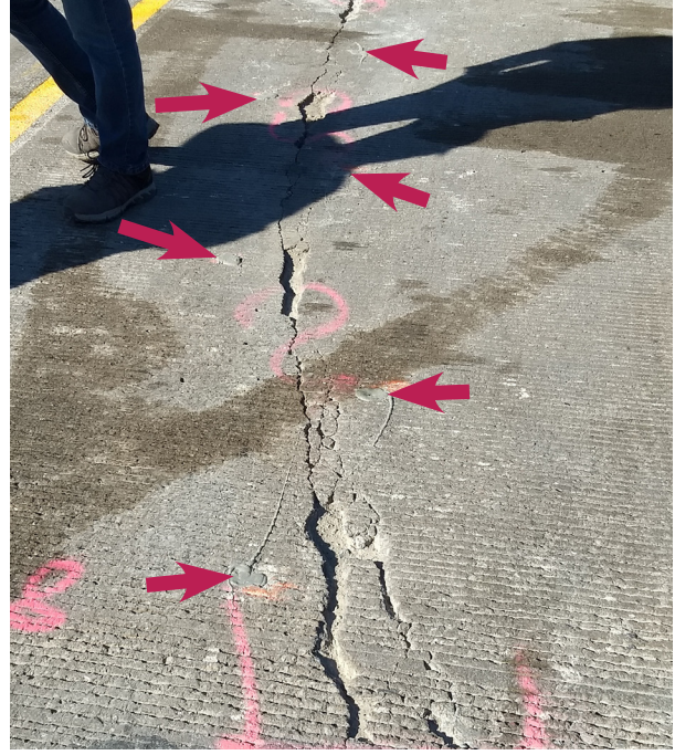
B. Completed cross-stitch repair (photo taken near SL28B00163L)
