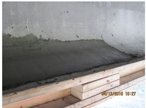
F. Finished Grout
