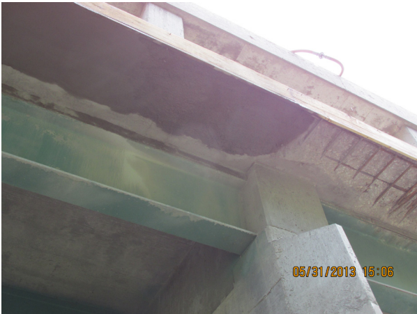
Figure 7.32—Concrete Patching at Deck Edges, with Shotcrete
