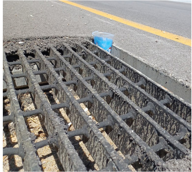
B. Shoulder Drain With Frame After Overlay
