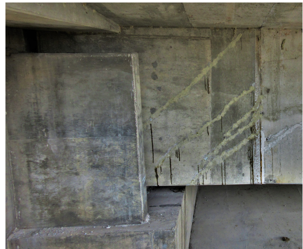
Figure 7.42—Crack Epoxy Injection on S002 50816
