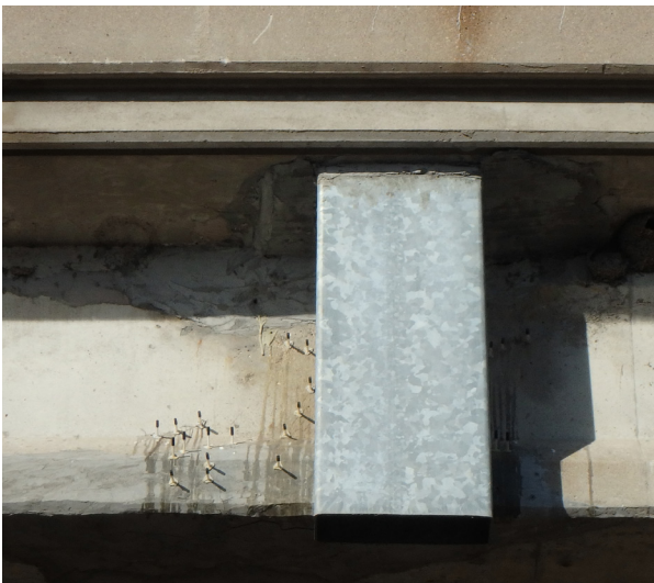
Figure 7.41—Crack Epoxy Injection on S070 10755
