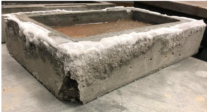
Figure 17 - A corner broke off of B7 during F-T testing. The block also exhibited a high degree of deposits.
