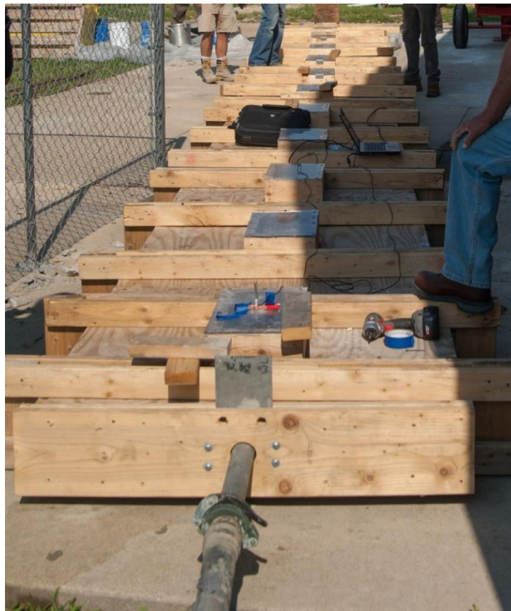
Figure 2.12 – Photo of the second pumping stage
