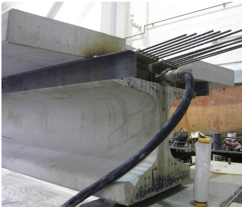
Figure 2.27 – Pumping concrete from the other end of the specimen
