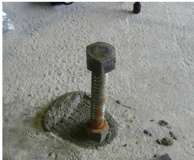
Figure 2.25 – Plugging 1 in. diameter vents
