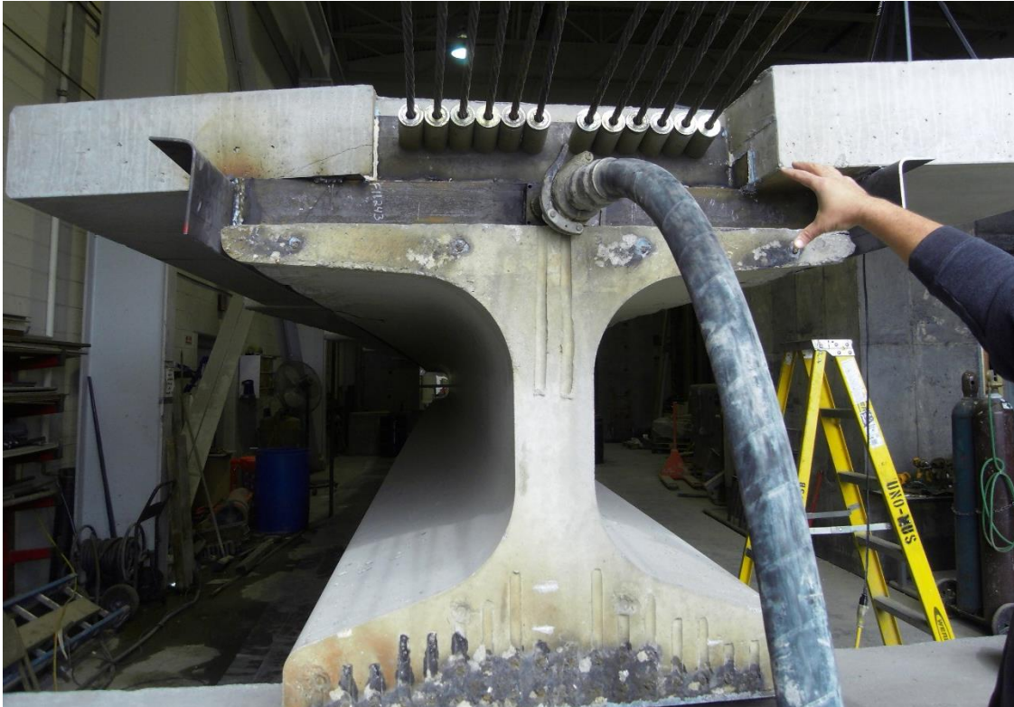
Figure 2.24 – Pumping SCC using 2 in. diameter hose
