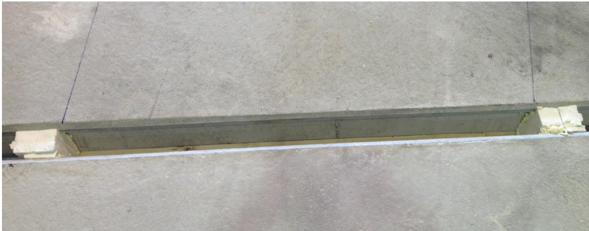
Figure 2.20 – Transverse joint between adjacent deck panels.
