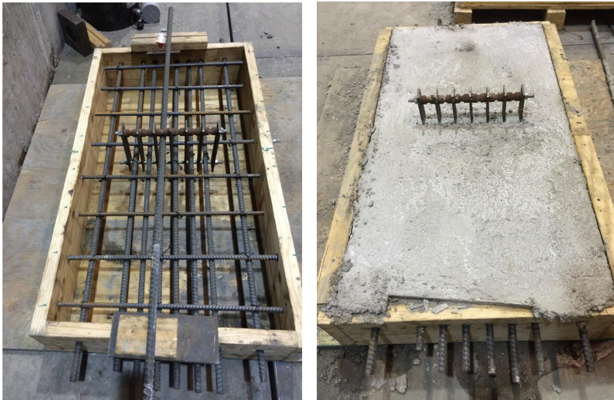
Figure 4.5: Specimen photos before and after concrete placement
