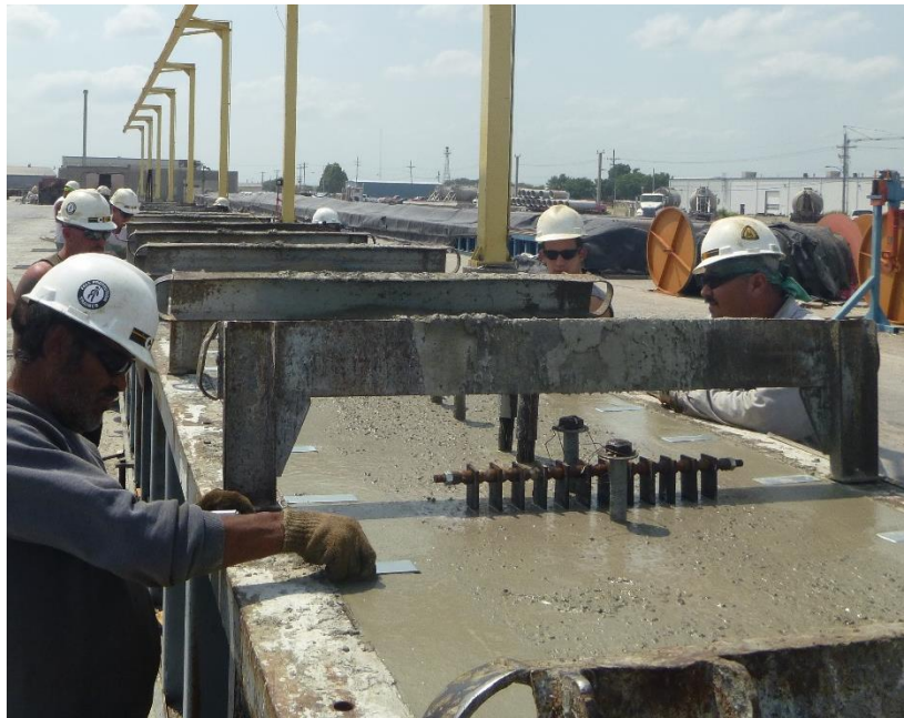
Figure 2.16 – Photos of girder fabrication
