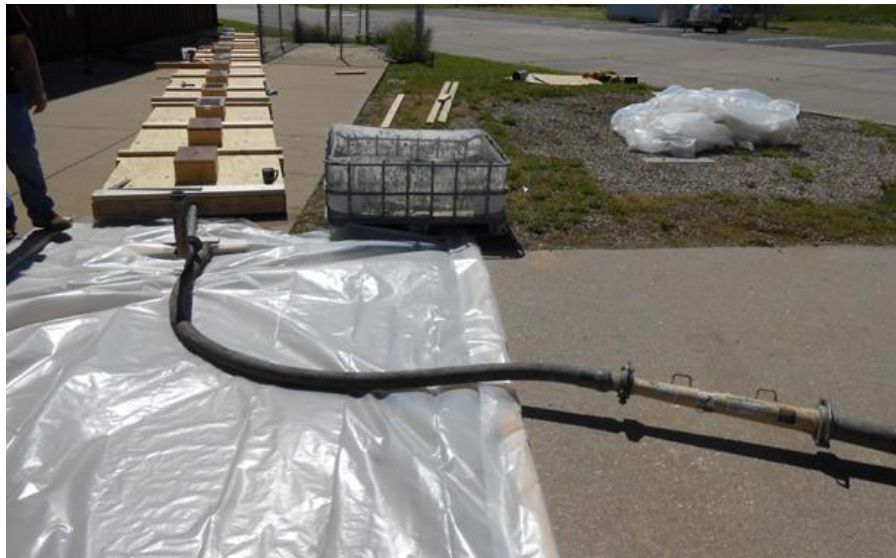
Figure 2.1 – Photo of the formwork and pump connection at one end
