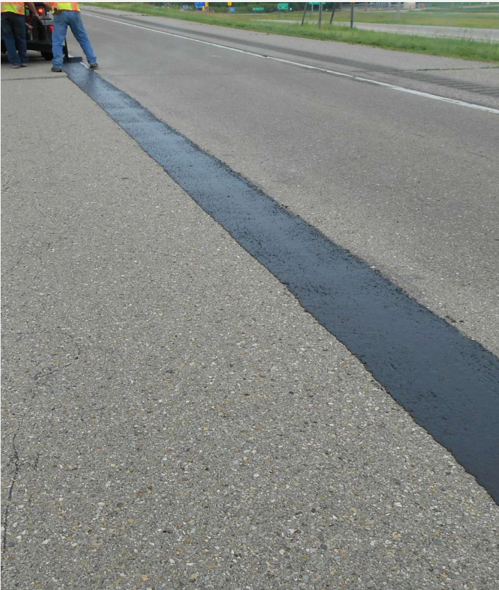
Repairing Deteriorated Longitudinal Joints
