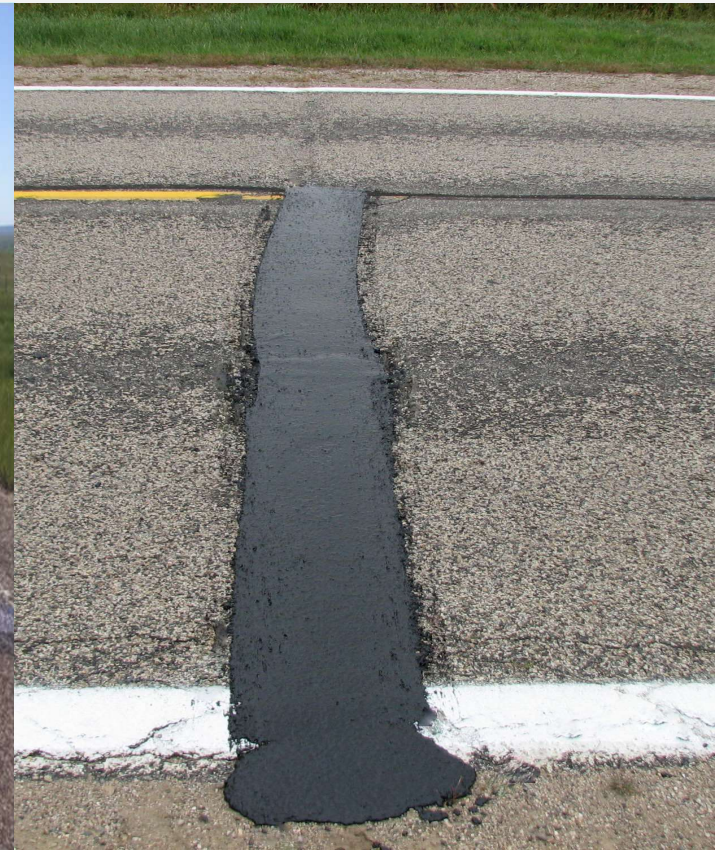
Filling Wide Cracks and Joints
