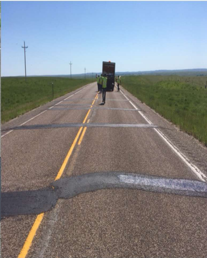
Leveling Depressed Thermal Cracks
